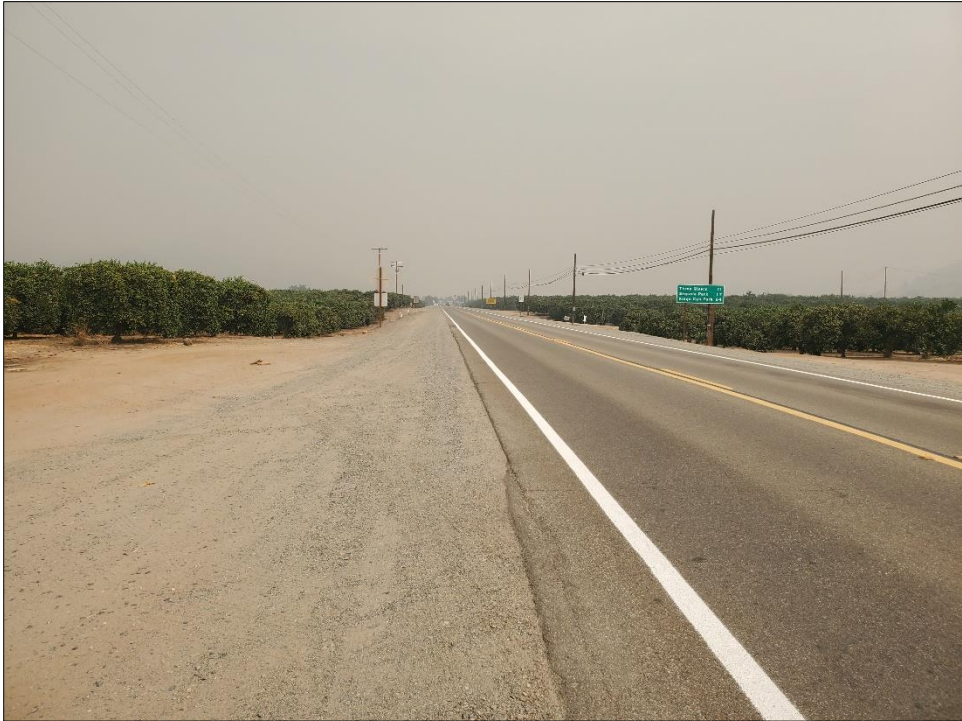
Photo 3: Pipeline alignment along SR 198 looking north.
