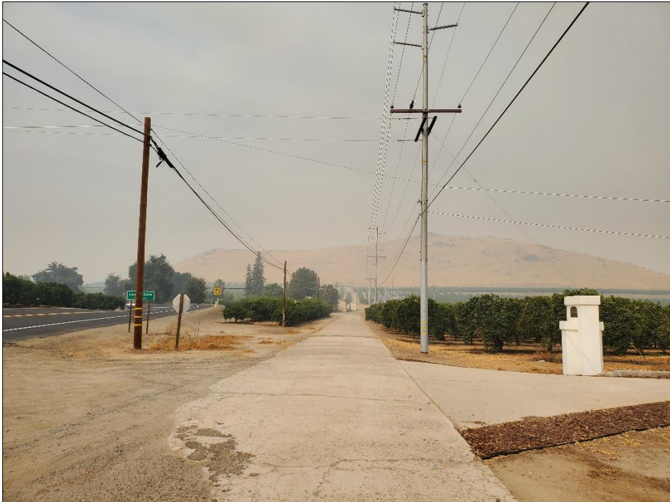
Photo 4: Pipeline alignment along Avenue 330 looking west.
