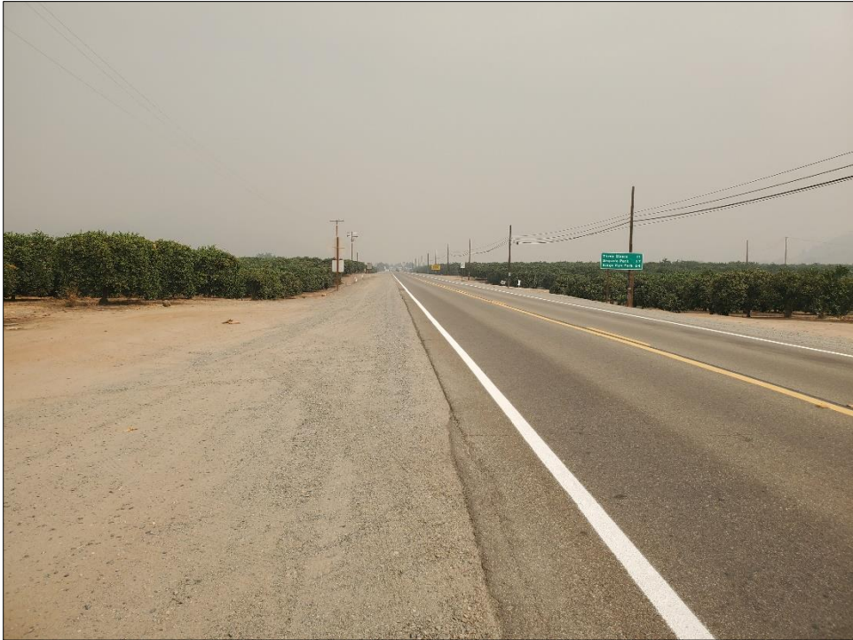
Photo 3: Pipeline alignment along SR 198 looking north.
