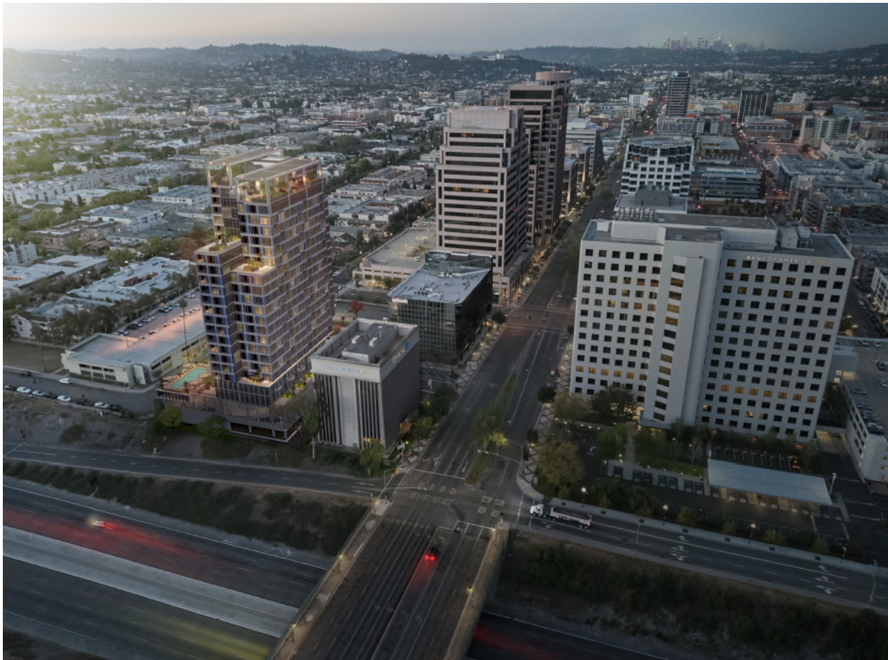
Figure 17: Aerial view looking south at intersection of the 134 Freeway and Brand Boulevard with the historic building and proposed new building on left (John Friedman and Alice Kimm Architects, 2021)
