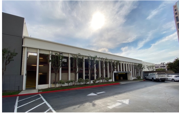
Figure 13: View looking southeast at west façade of parking structure (TGHP, September 2021)
