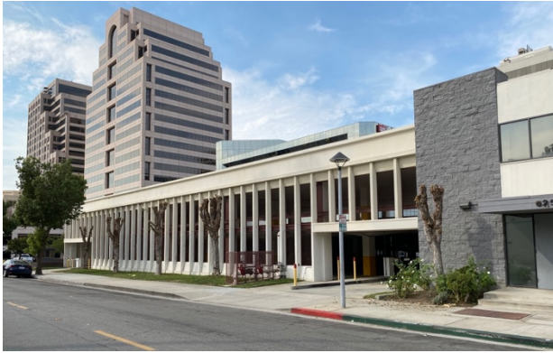
Figure 12: View looking southwest at east façade of parking structure (TGHP, September 2021)
