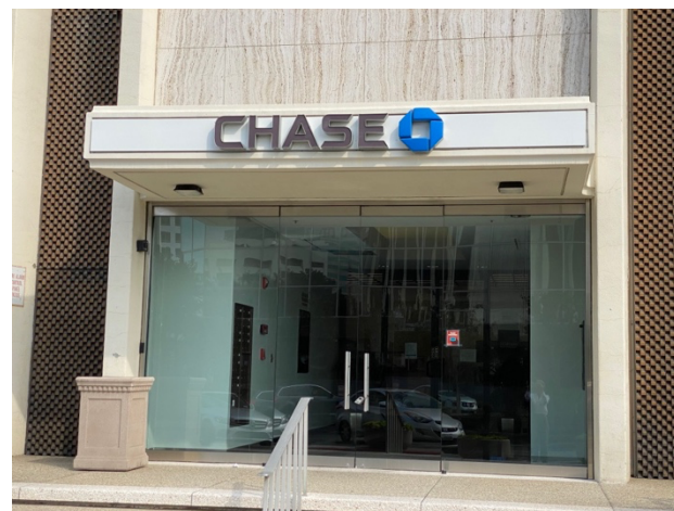
Figure 11: View looking north at entrance on south façade of office building (TGHP, September 2021)
