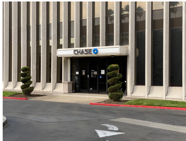
Figure 9: View looking southwest at entrance on east façade of office building (TGHP, September 2021)
