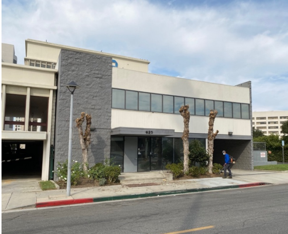
Figure 14: View looking northwest at east façade (TGHP, September 2021)
