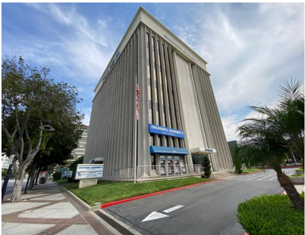
Figure 8: View looking northeast at south and west elevations of office building (TGHP September 2021)
