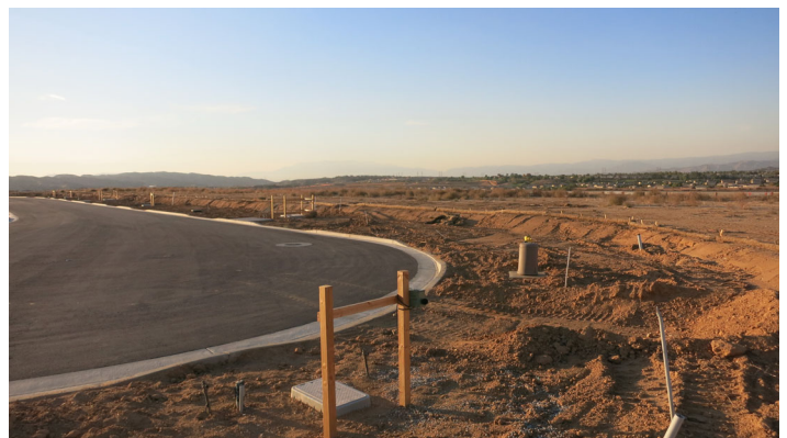
Noise Measurement Site B - looking northwest
