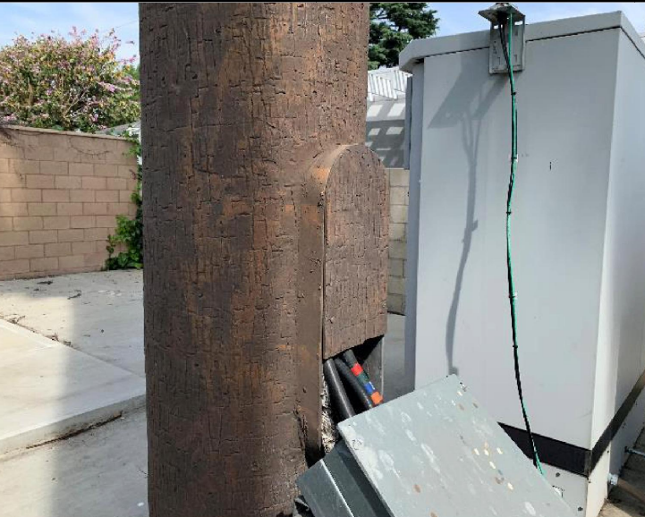
View of Inside Cell Site Panoramic #5
