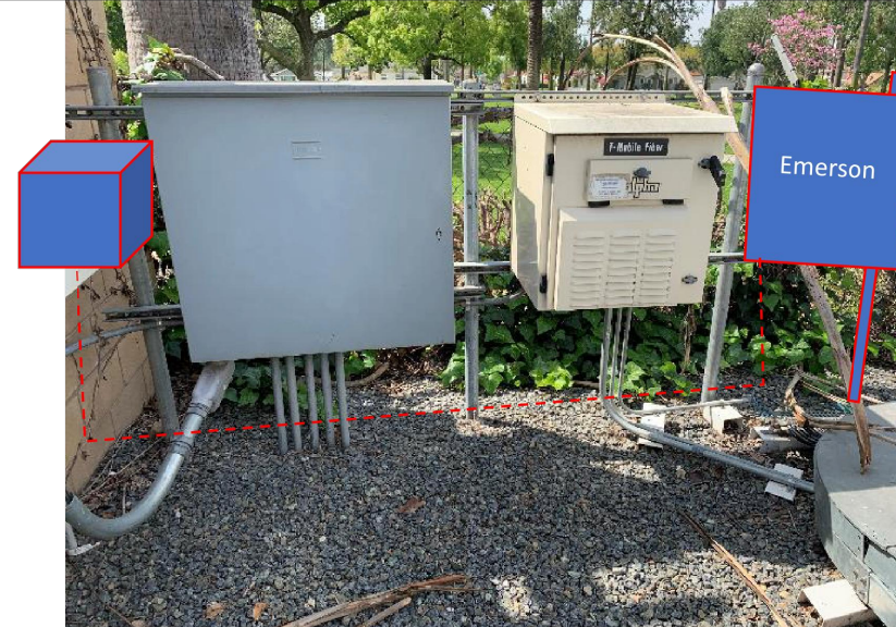
View of (N) 2" Telco Conduit from the (N) Telco Cabinet to the (N) AAV Cabinet
