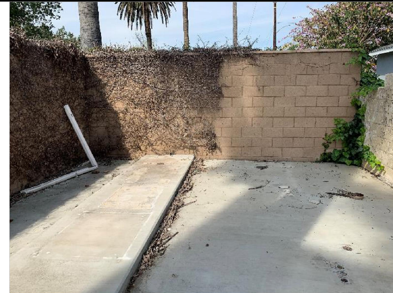
View of Inside Cell Site Panoramic #2
