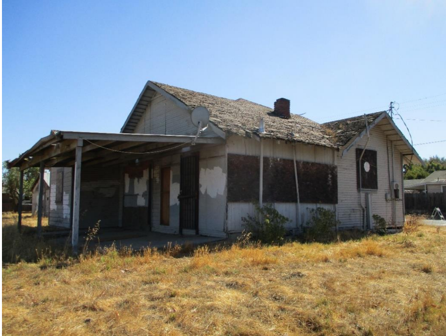
Figure 3. West elevation, facing southeast.
