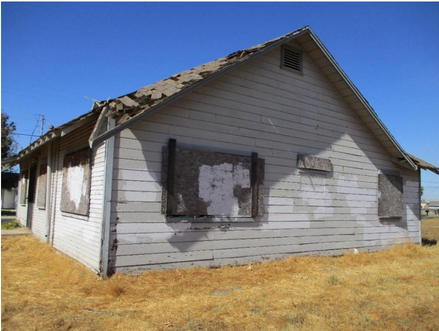
Figure 8. East elevation, facing northwest.
