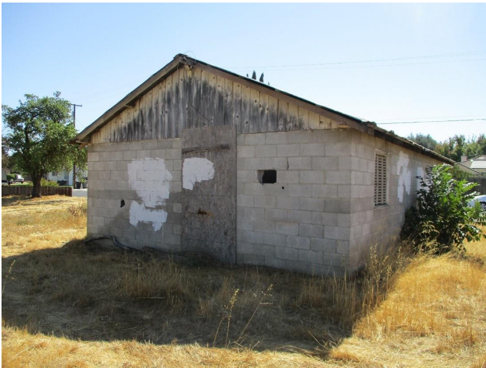
Figure 43. North elevation, facing south.
