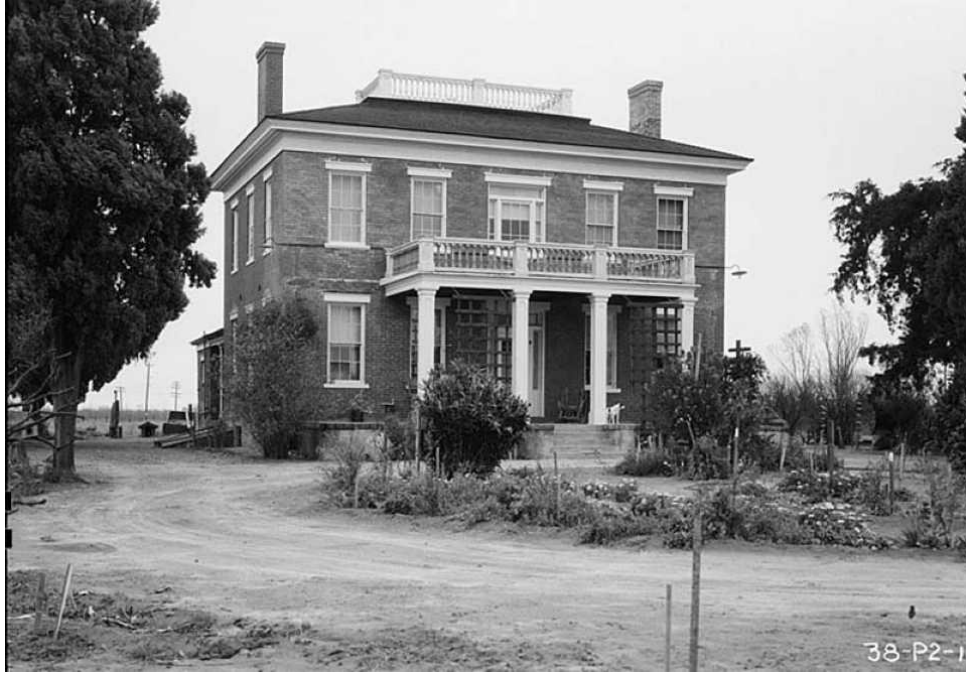
Figure 13. John Wheeler Jones' 1867 two-story brick house (extant) along French Camp Road in Escalon (courtesy of Library of Congress). 50
