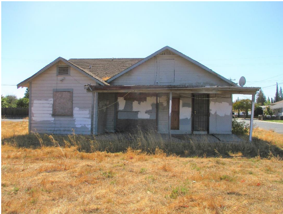
Figure 5. North elevation, facing west.
