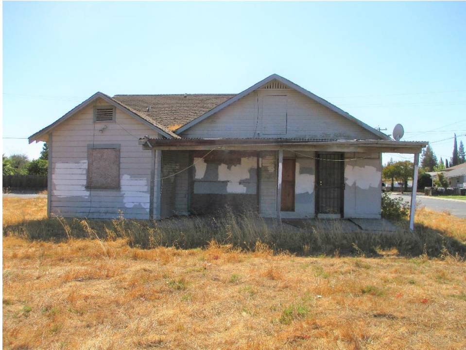
Figure 38. North elevation, facing west.
