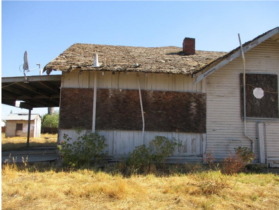
Figure 37. West elevation, showing the hipped gable form clad in vertical wood boards, facing east.
