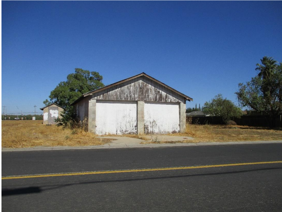
Figure 42. Photograph showing the primary façade (south elevation) of the ca. 1930 detached garage, facing north.
