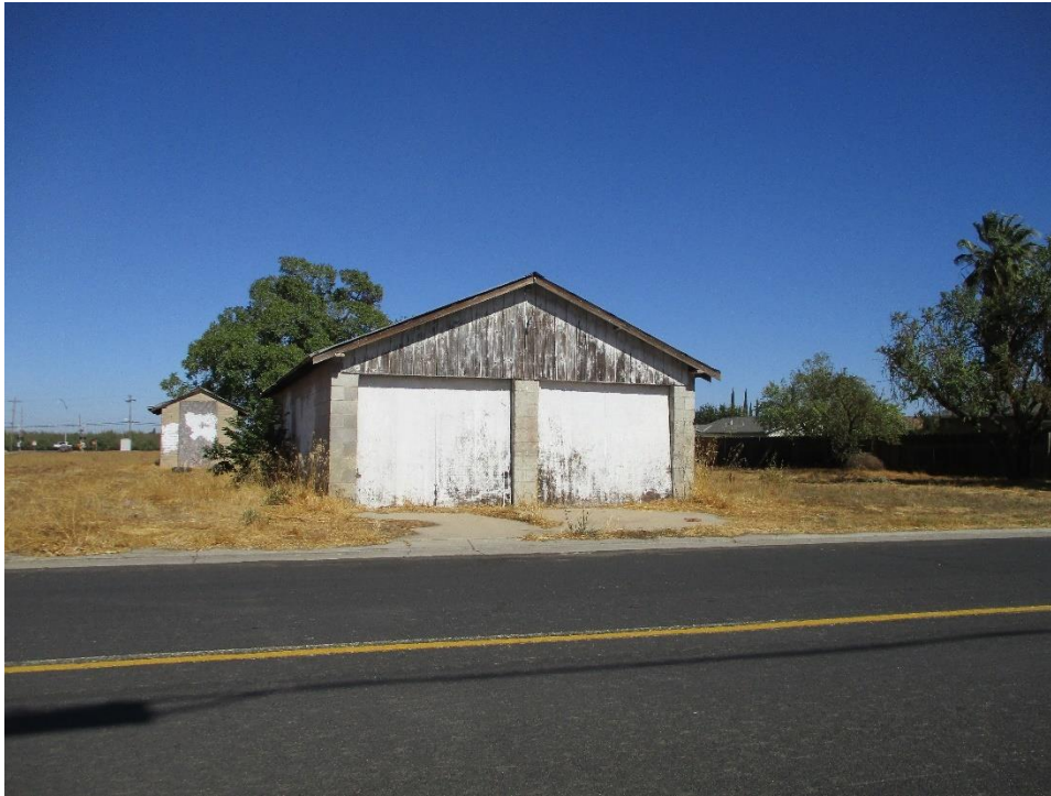
Figure 9. Photograph showing the primary façade (south elevation) of the ca. 1930 detached garage, facing north.
