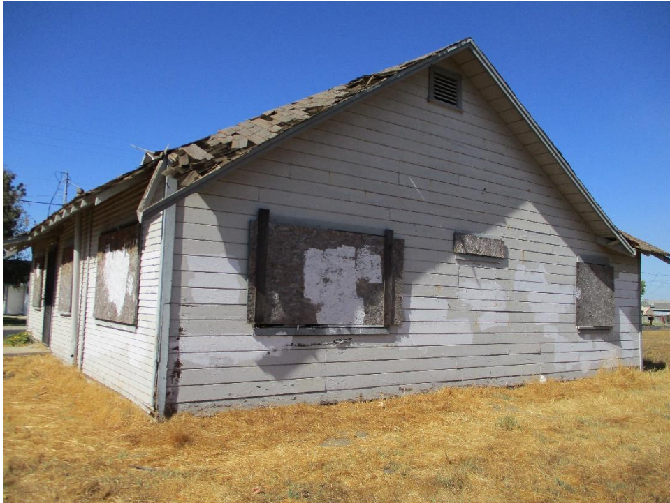
Figure 41. East elevation, facing northwest.
