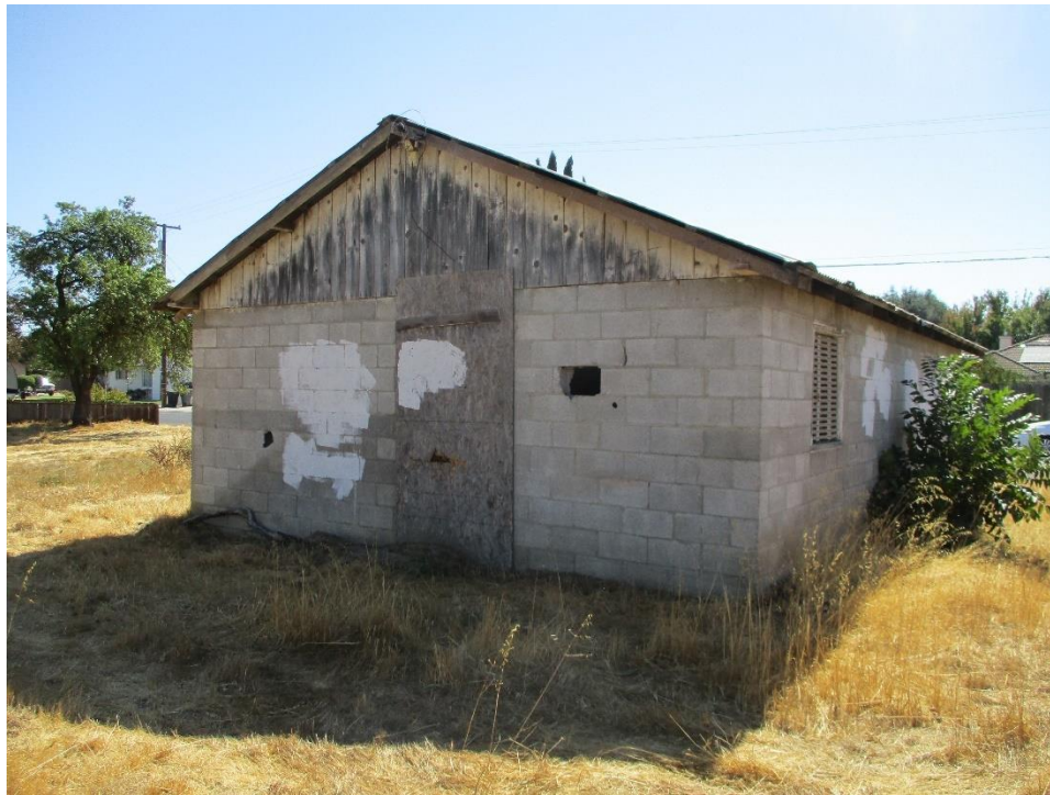
Figure 10. North elevation, facing south.
