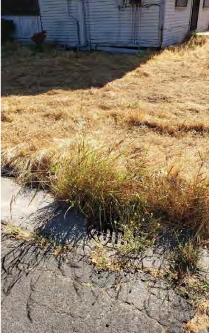
Photo 11: Storm sewer catch basin near southwest corner of APN 225-070-320.
