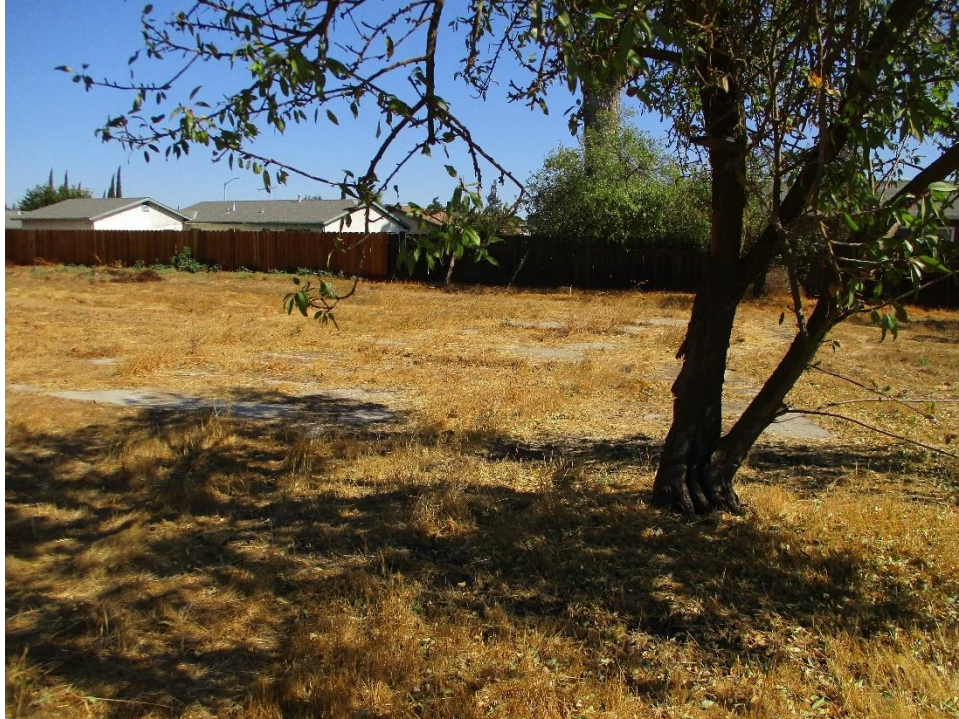
Figure 46. Photograph showing the concrete slab foundations and Almond tree (facing east).
