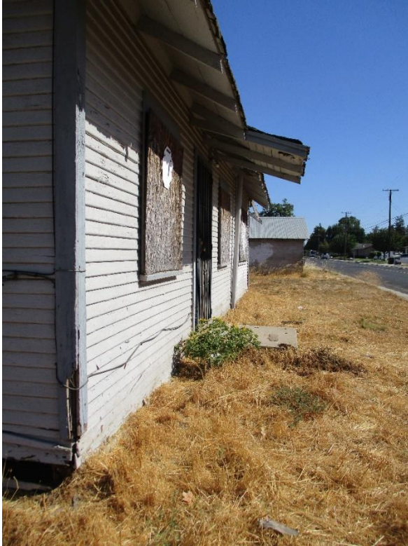
Figure 2. South elevation, facing east.
