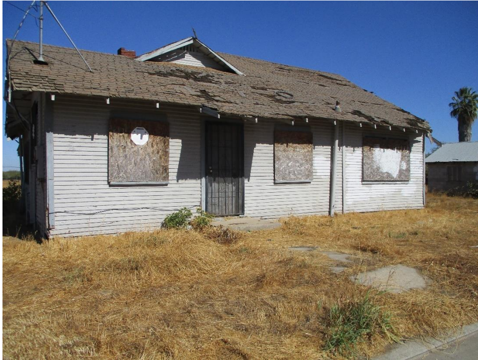
Figure 34. South elevation, facing northeast.
