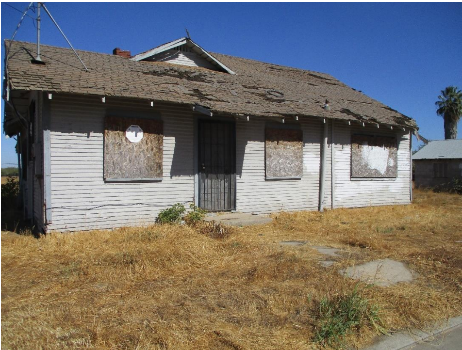
Figure 1. South elevation, facing northeast.
