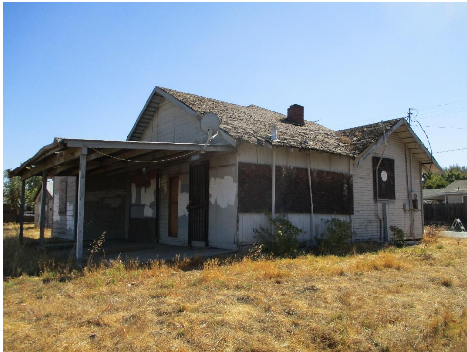
Figure 36. West elevation, facing southeast.
