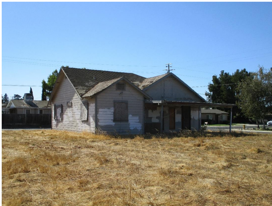
Figure 6. North elevation, showing the lower gable addition, facing south.
