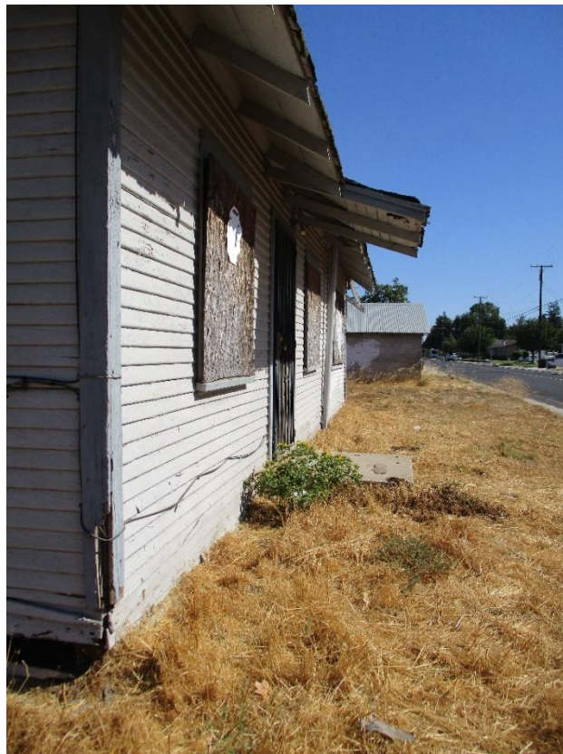
Figure 35. South elevation, facing east.
