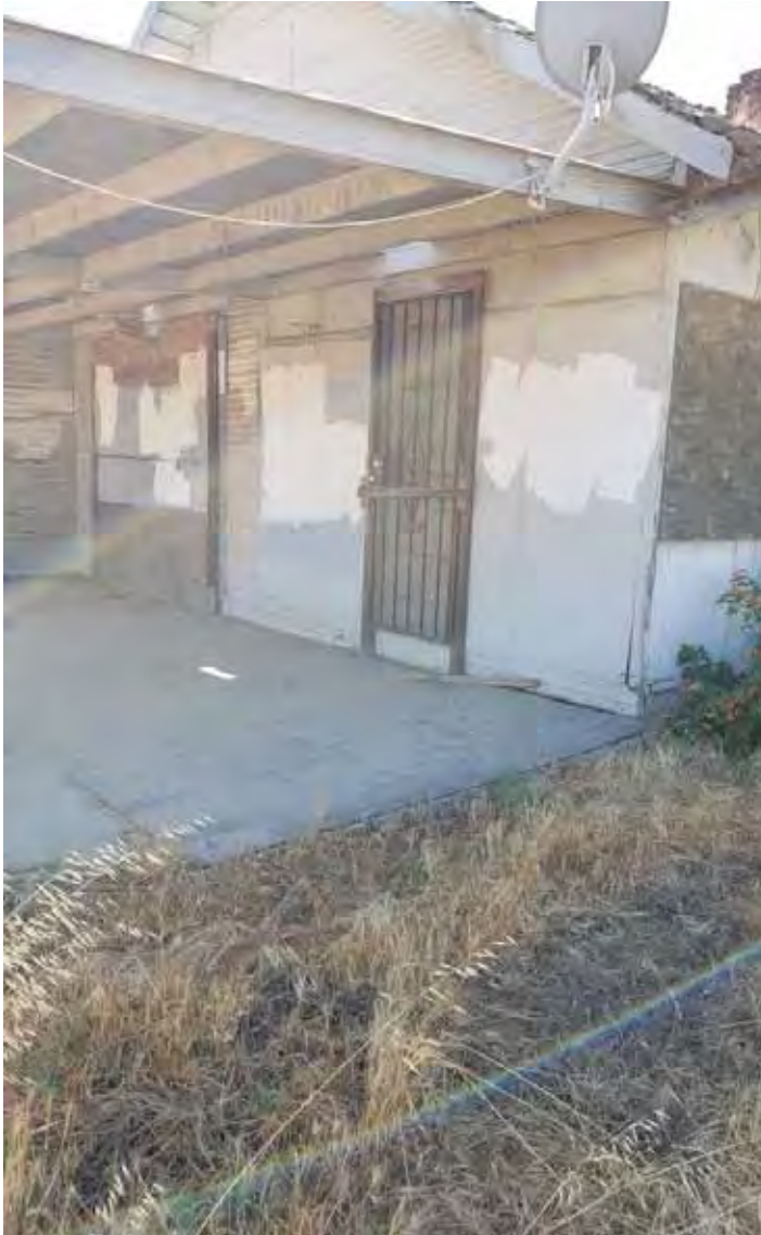
Photo 17: Rear of residence showing boarded up entrance to cellar.
