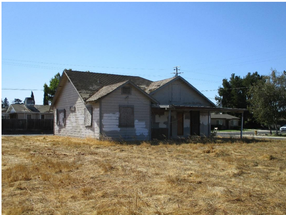
Figure 39. North elevation, showing the lower gable addition, facing south.
