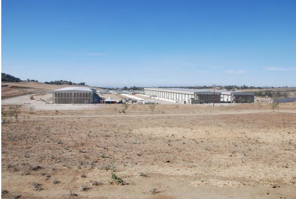
Photograph 1 – Overview of the proposed manure processing facility site, facing west-northwest.
