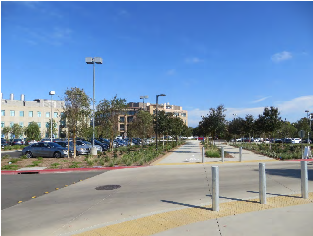
Photograph 10: Standing to the southwest of the project site, facing northeast.
