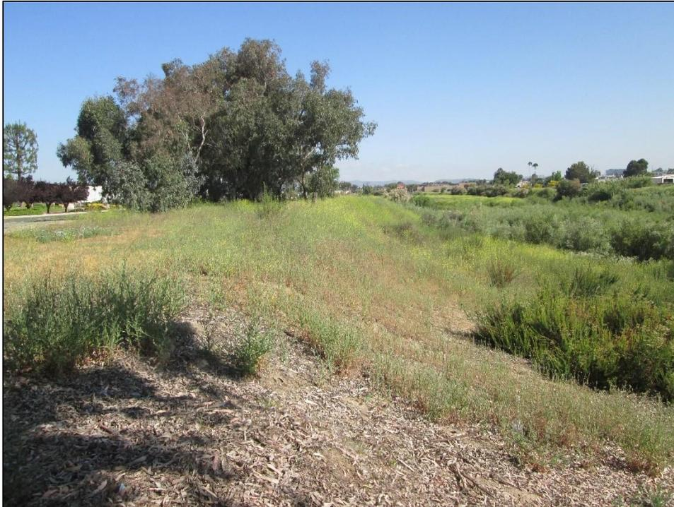
Figure 8. Earthen channel bank slope exposing pockets of Holocene- to late Pleistocene-age young alluvial valley deposits (Qyva), consisting primarily of sands. View facing to the north.
