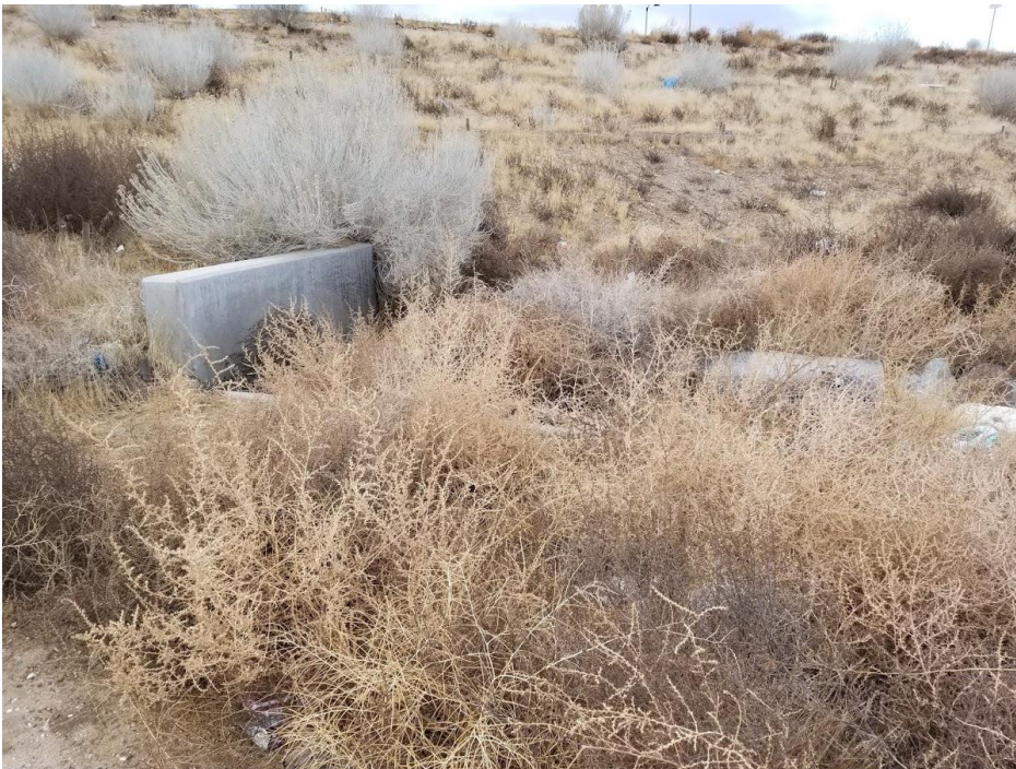
Photo 4: storm drain culverts (view W)
