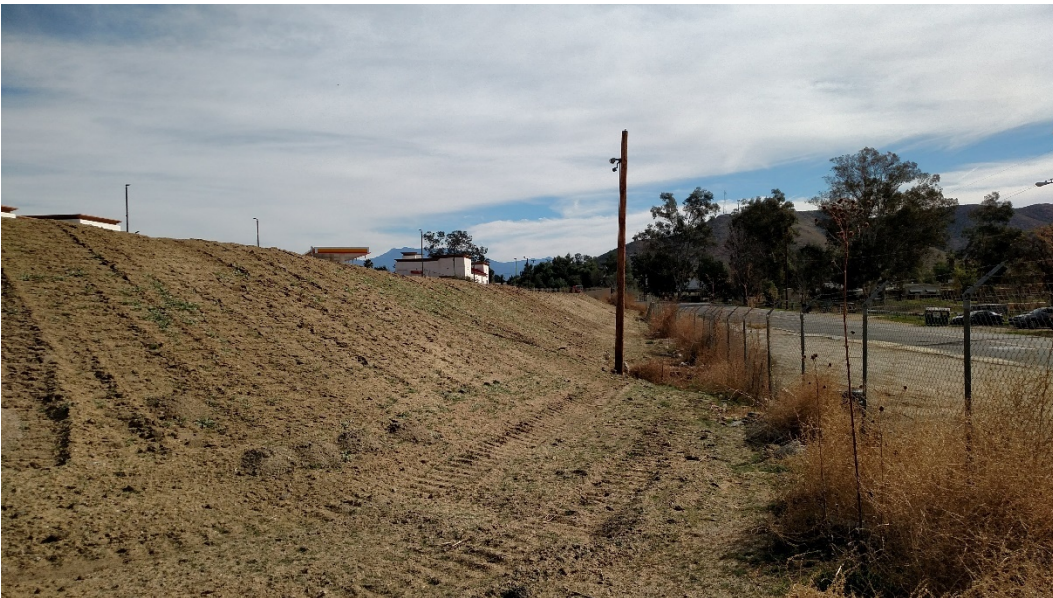
Figure 8. View of southwestern portion of project site, facing east.
