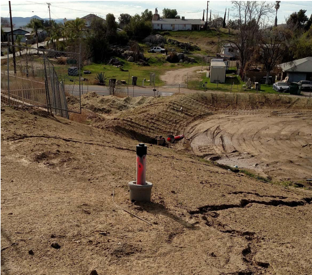
Figure 6. View of portion of project site apparent sewer installation, facing south.
