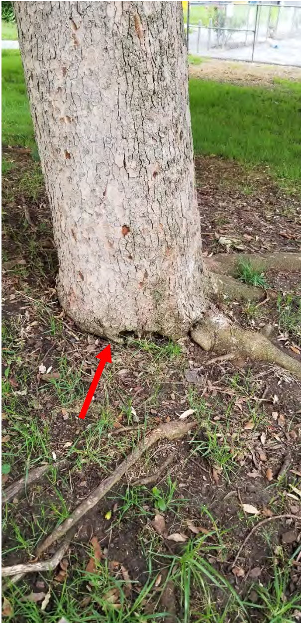
Figure 3: Evidence of girdling root on tree #8 shown by red arrow.
