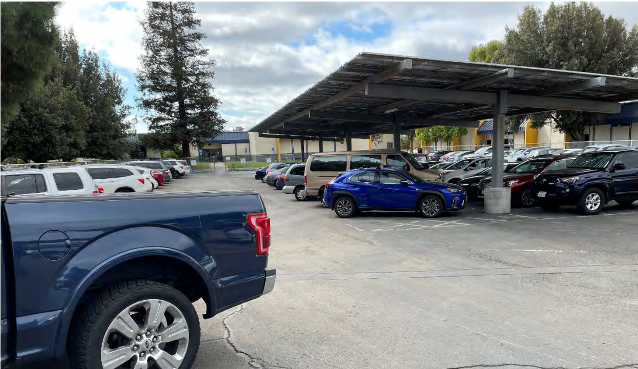
3. Existing parking/solar canopy area where PAC would be located looking south
