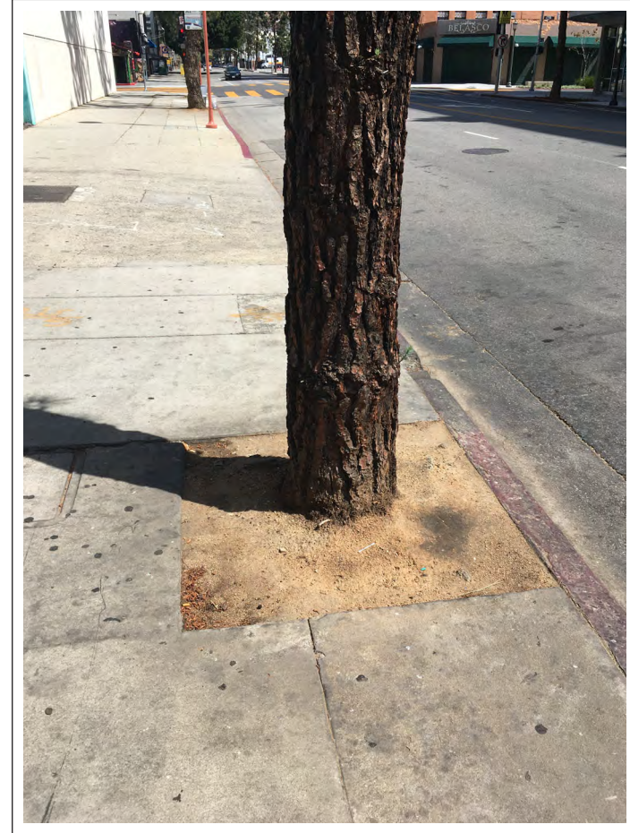
March 28, 2020. View of base of Tree 1. Tree is not causing any damage to sidewalk or curb.
