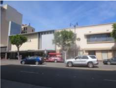
NORTH ADJACENT SITES LOOKING NORTHWEST FROM THE NORTHEAST SUBJECT PROPERTY CORNER
