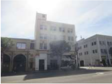
SUBJECT PROPERTY LOOKING SOUTH FROM HOLLYWOOD BOULEVARD
