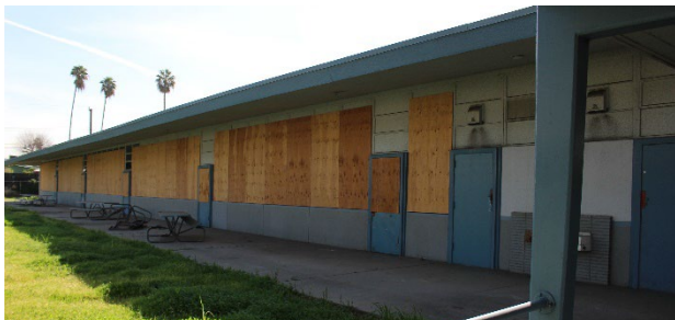
Figure 12: Building F. South elevation above and north elevation below. 2020. Source: GPA.
