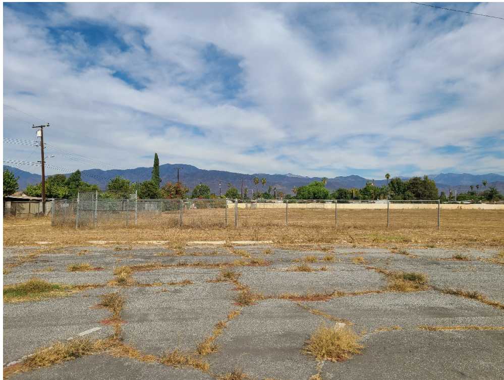
Photograph 1: Overview of the former field and baseball diamonds located behind Griswold School passed the deteriorated parking lot, facing north.
