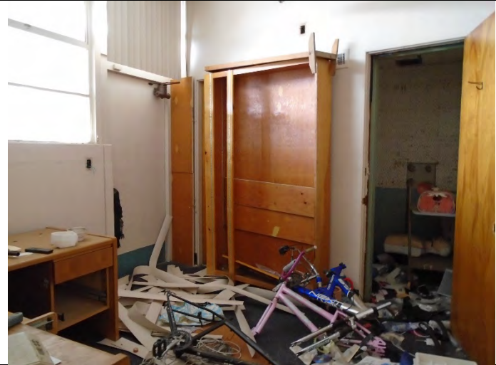
Typical administration office interior
