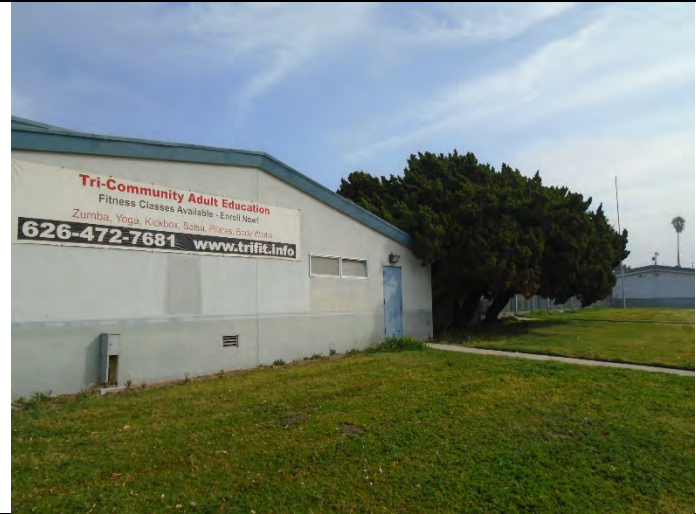
Typical building exterior
