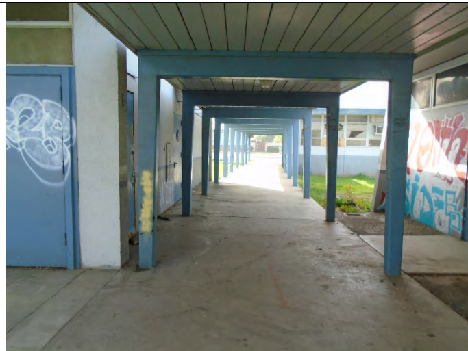
Typical building exterior
