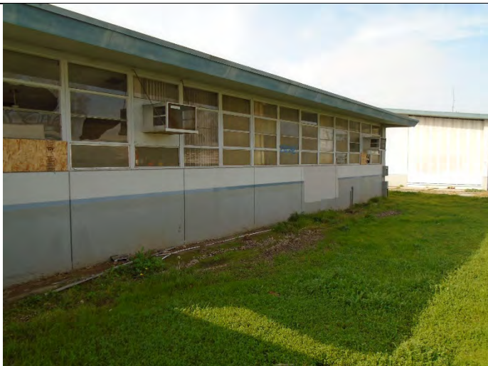
Typical building exterior
