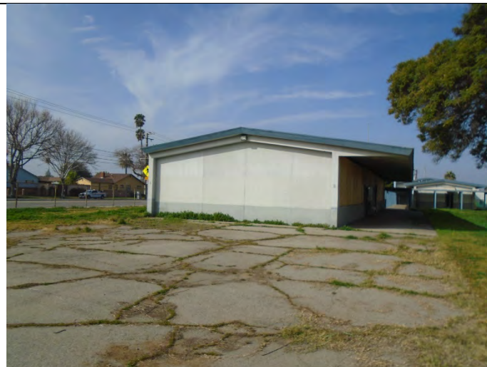
Typical building exterior
