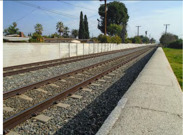
View Northeast toward adjoining residential properties
