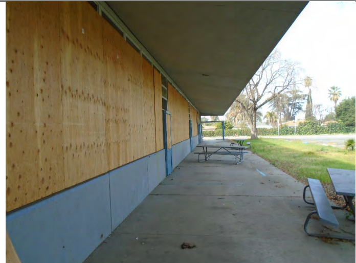
Typical building exterior
