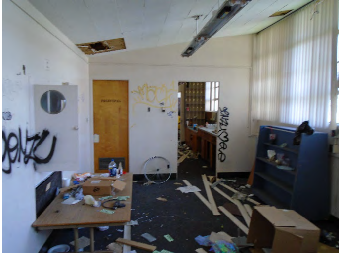
Typical administration office interior
