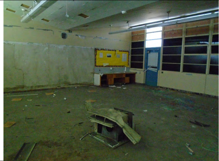
Typical classroom interior
