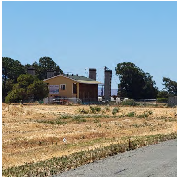
Photograph 2-2 Existing Algae Facility on Project Site
