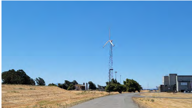
Photograph 2-8 View Looking South at Project Site and Existing Windmills
