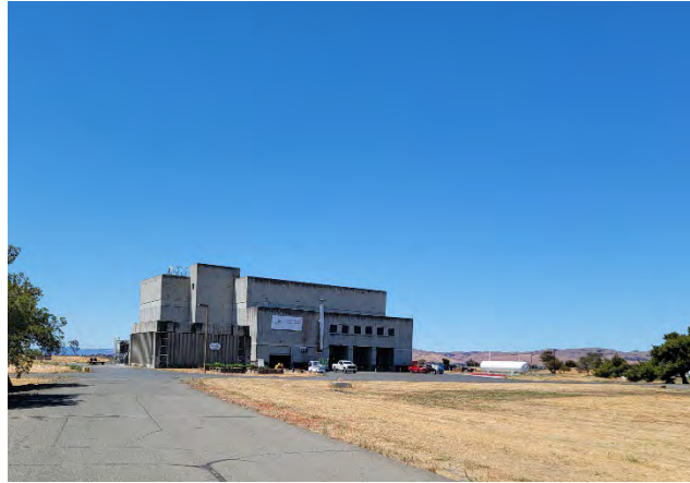
Photograph 2-1 Dewatering Building and Organic Materials Recovery Center
