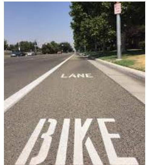
Figure 11. Dedicated Bicycle Facilities Can Improve Safety and Comfort for People Riding
