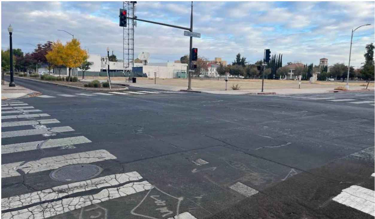
Figure 8 Stanislaus Street and Van Ness Avenue Intersection, Facing North
