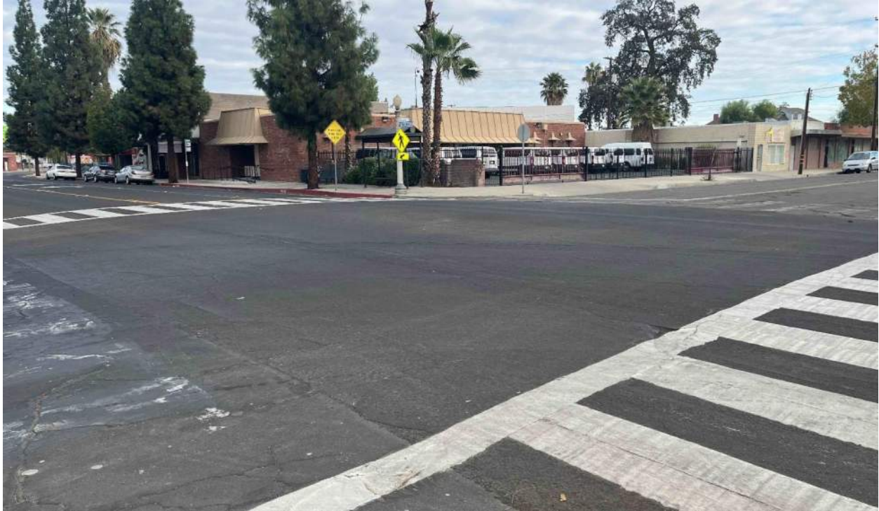
Figure 5 Intersection of Van Ness Avenue and Amador Street, Facing North
