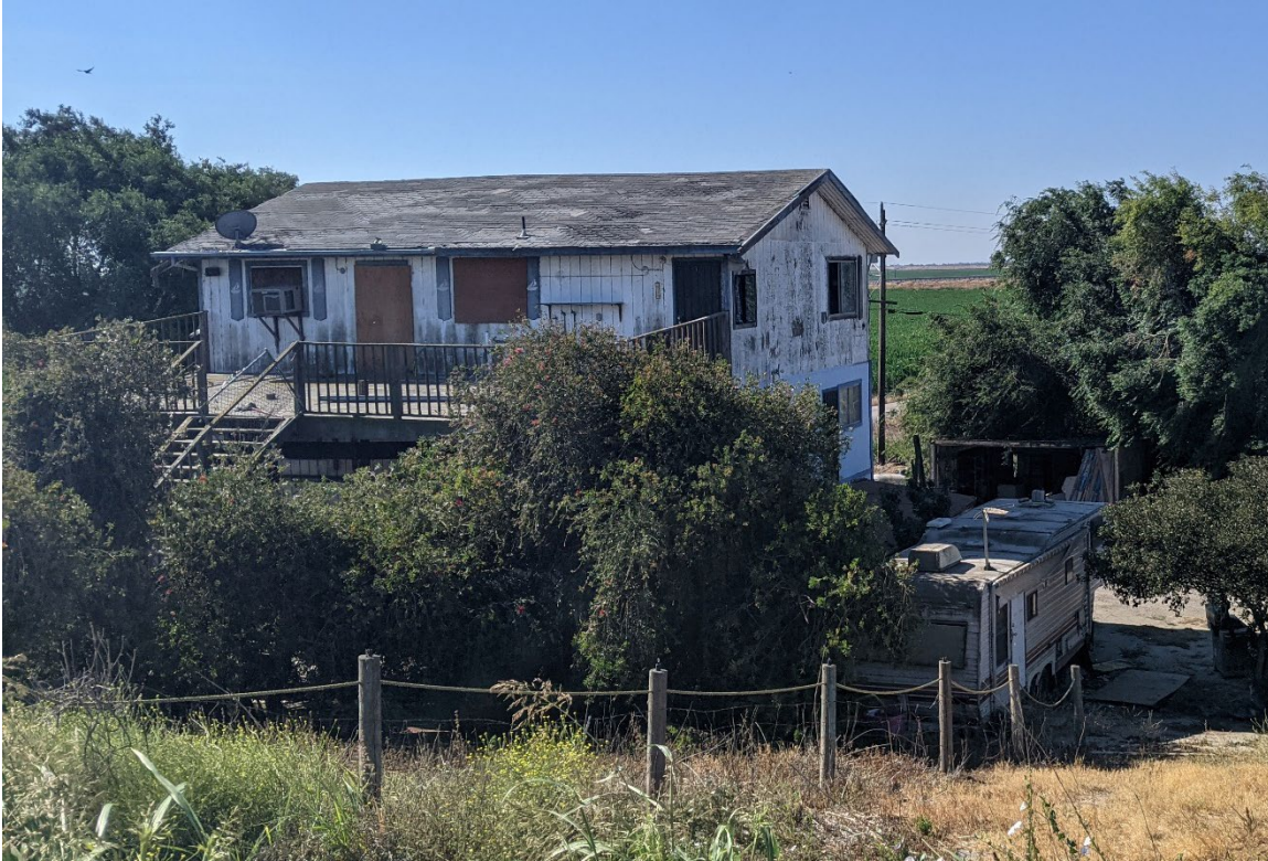
Figure 1-4. Uninhabited residence at levee station 824+50 to be demolished as part of the Bouldin Island Levee Rehabilitation Project.
