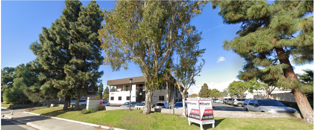
Northwestern views of the southern boundary of the Project Site from Slater Avenue.
