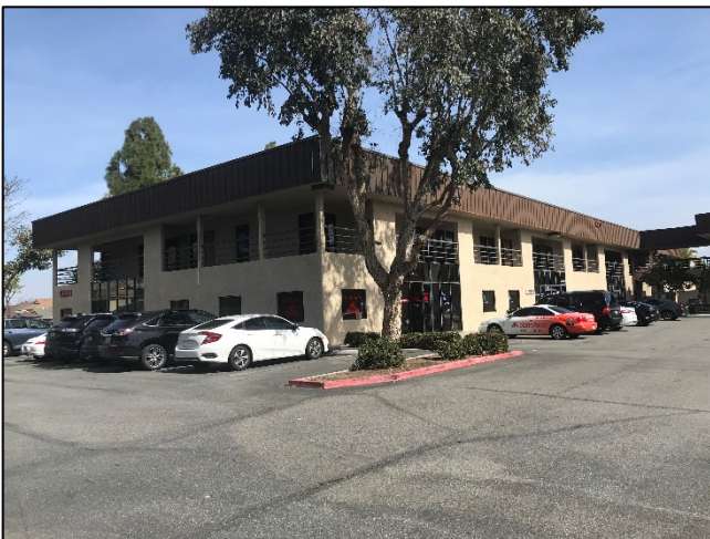
Figure 36. Overview of modern office building, facing northeast
