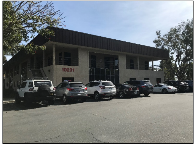
Figure 35. Overview of modern office building, facing northeast
