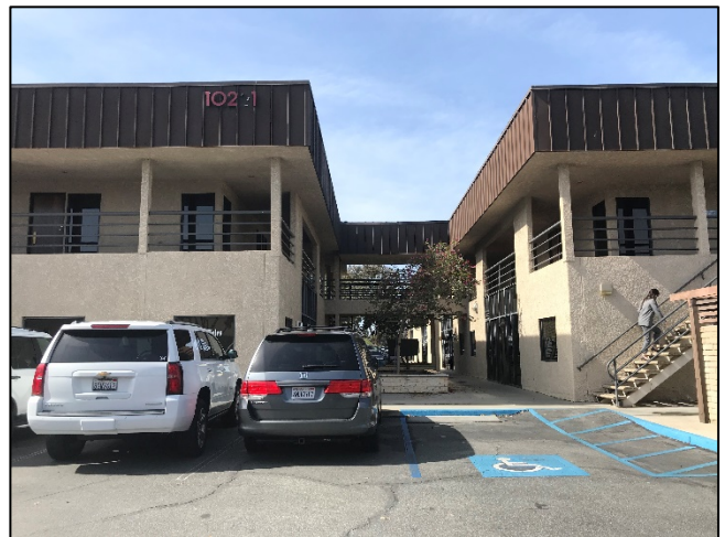
Figure 37. Overview of modern office building, facing west
