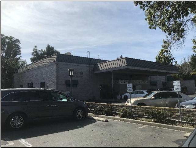
Figure 34. Overview of backside of restaurant at 10201 Slater Avenue, facing southwest
