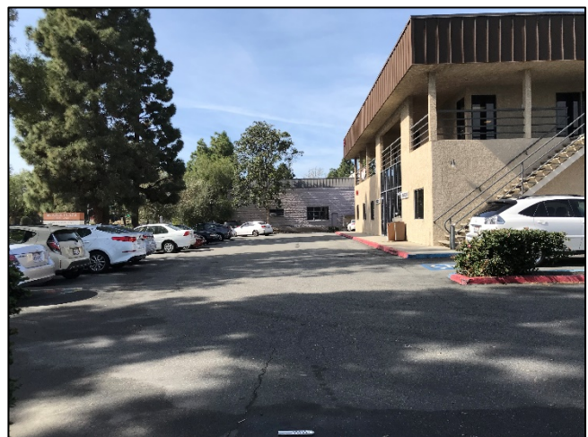
Figure 21. Overview of Project Area from southeast corner, facing west
