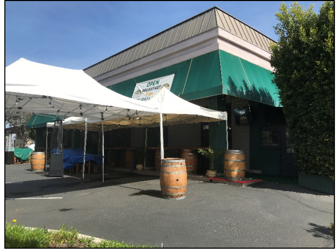
Figure 31. Overview of restaurant at 10201 Slater Avenue, facing northeast
