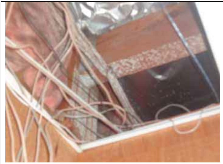
29. Example of the wood framed roof structure.
