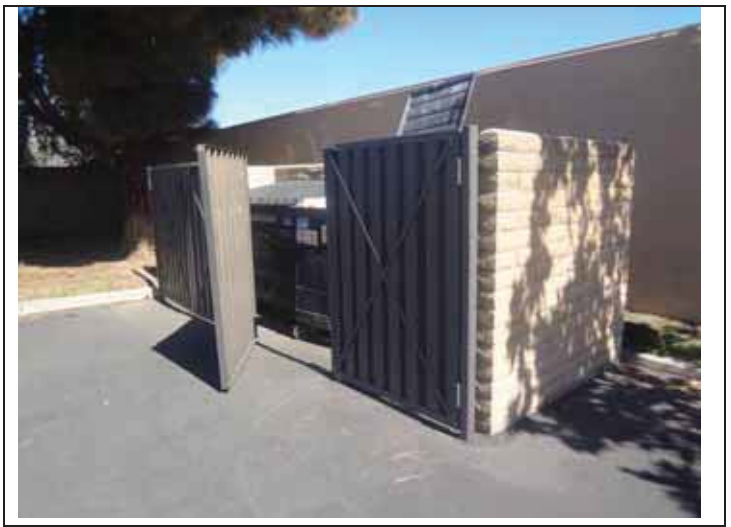
26. On-site solid waste trash enclosure.
