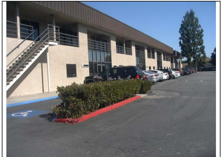
4. View of east side of 10221 building.
