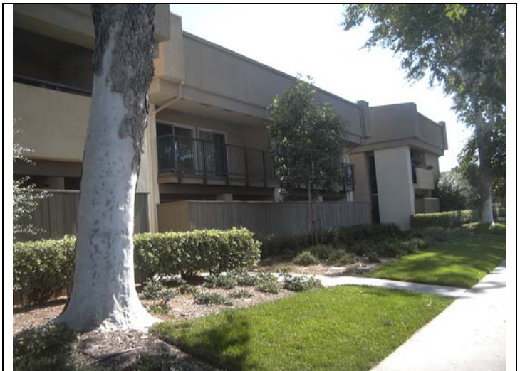
24. View of an apartment complex immediately east.
