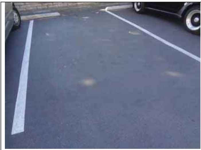
17. Typical asphalt pavement and parking stall striping condition.
