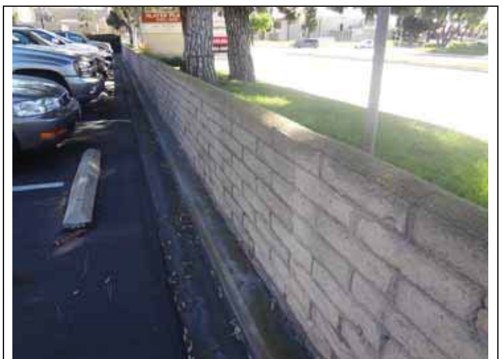
12. Concrete masonry retaining wall along the front property line.
