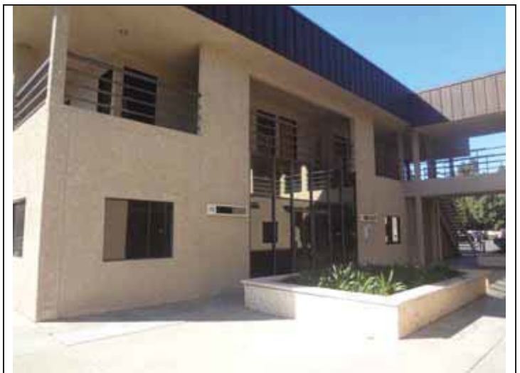
4. North elevation of the 10221 Building.
