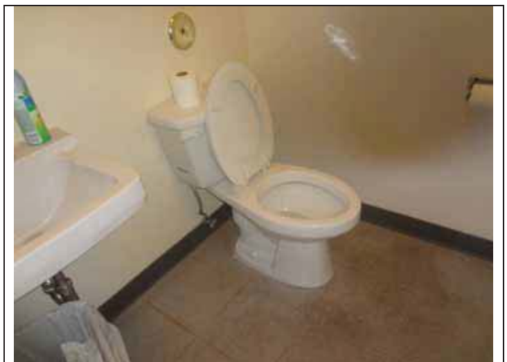
66. Private restroom within one of the tenant spaces.
