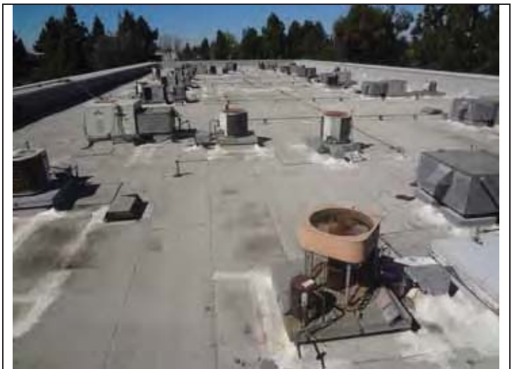
32. The 10231 Building roof.
