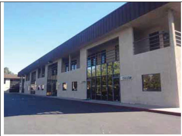
3. West elevation of the 10221 Building.
