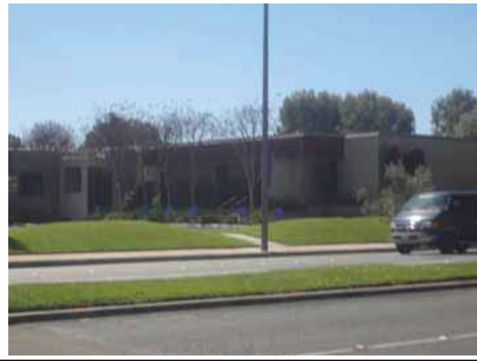
73. Adjacent property south of the subject property, across Slater Avenue.
