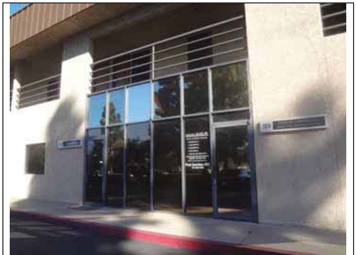
38. Typical ground floor storefront system and tenant space entrance.
