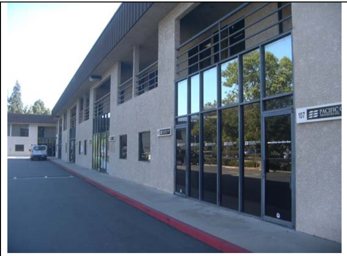
3. View of west side of 10221 building.
