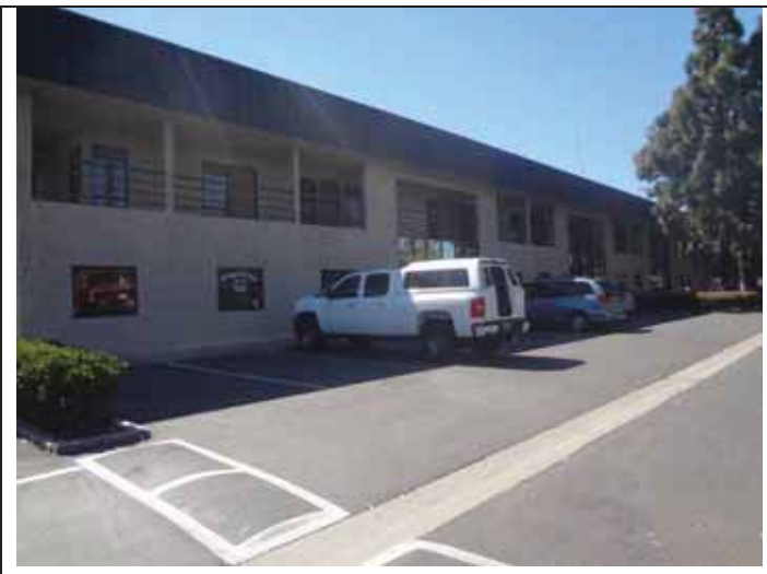
7. North elevation of the 10231 Building.
