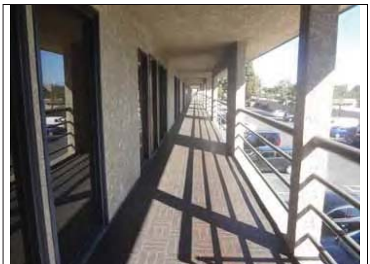
42. Typical second floor walkway.
