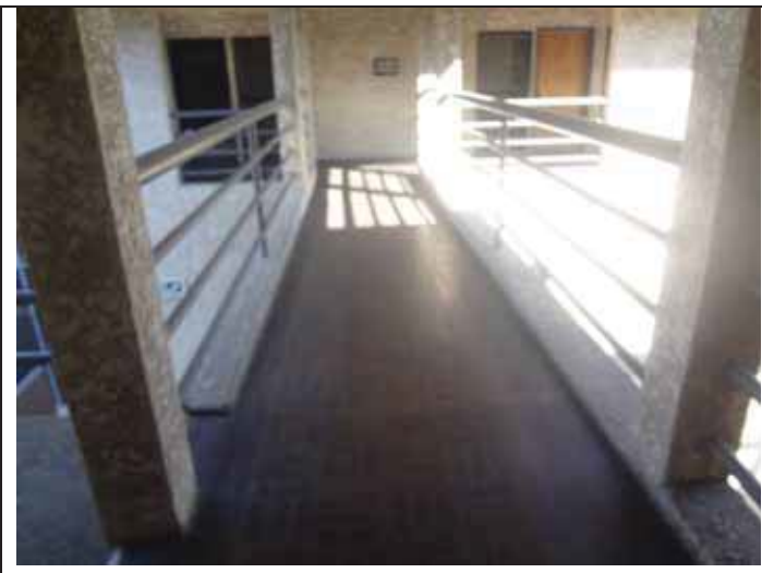
43. Pedestrian bridge connecting the two buildings.
