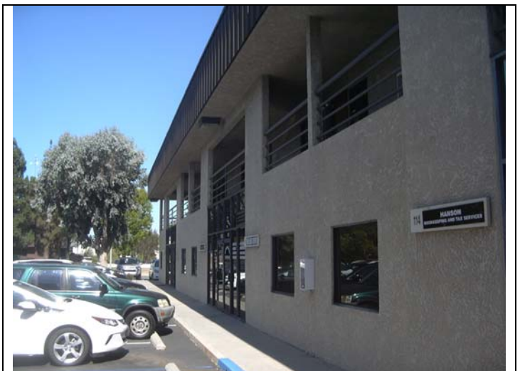
12. View of south side of 10231 building.
