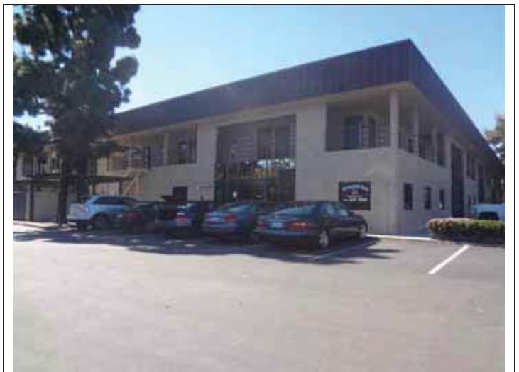
8. East elevation of the 10231 Building.
