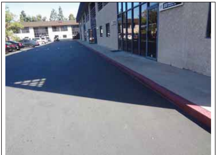
18. Typical raised concrete pedestrian walkway that runs along the perimeter of the buildings.
