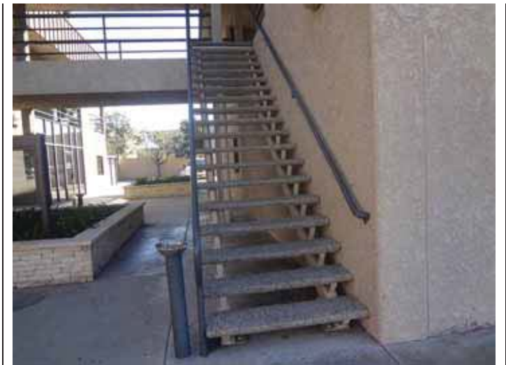
68. Stairways with open risers.
