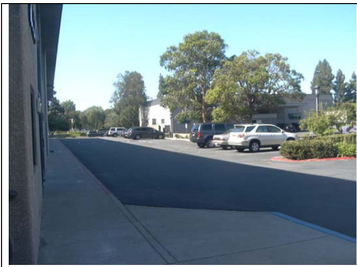
11. View of west portion of the subject property.
