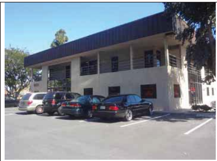
9. West elevation of the 10231 Building.
