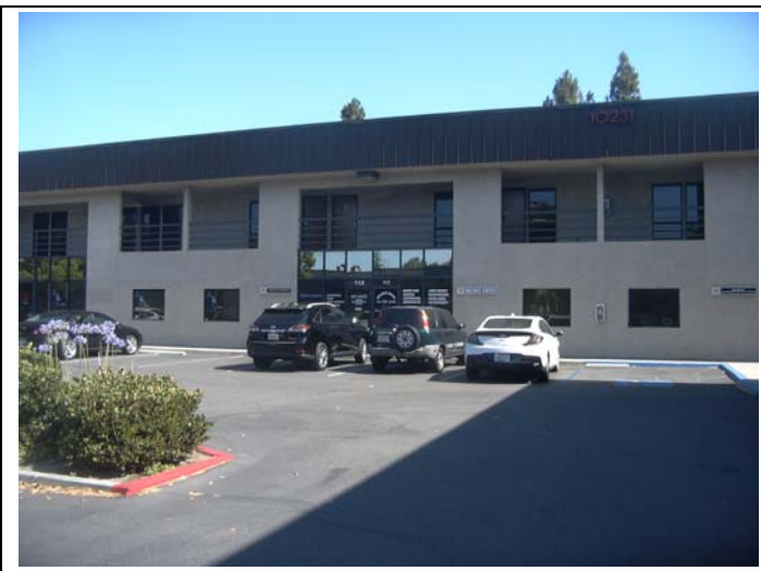
1. View of south side of 10231 building.
