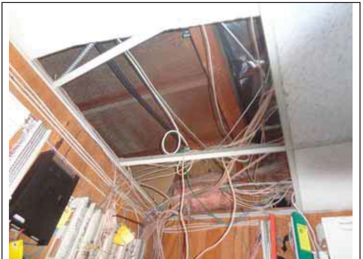
30. Example of the wood framed roof structure.
