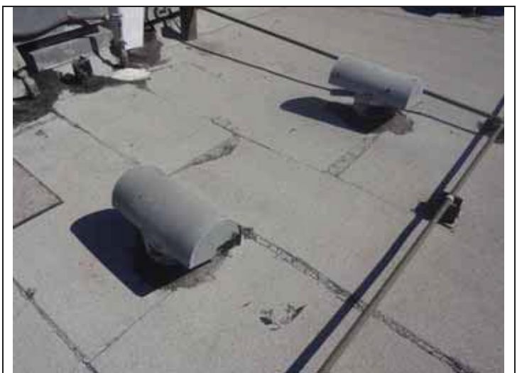
36. Typical roof vents.
