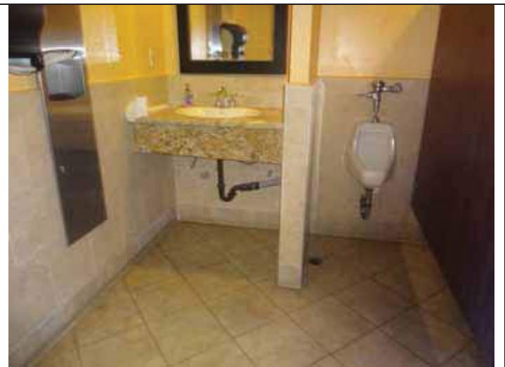
54. One of four common restrooms.
