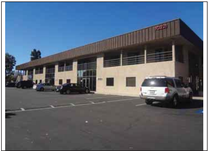
2. East elevation of the 10221 Building.
