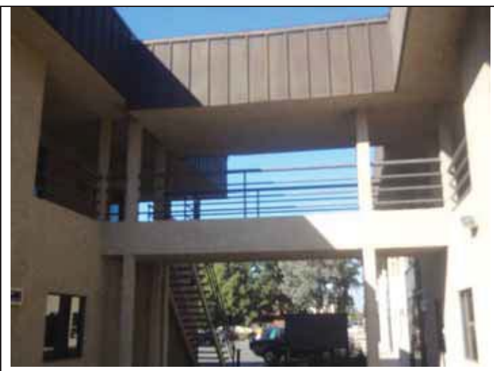
5. Pedestrian bridge connection the two buildings.
