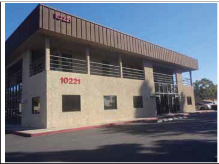
1. Front (south) elevation of the 10221 Building.
