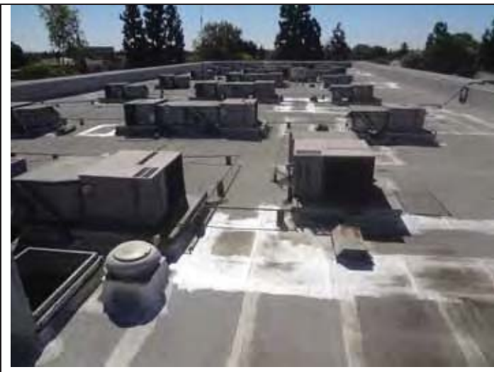
31. The 10221 Building roof.
