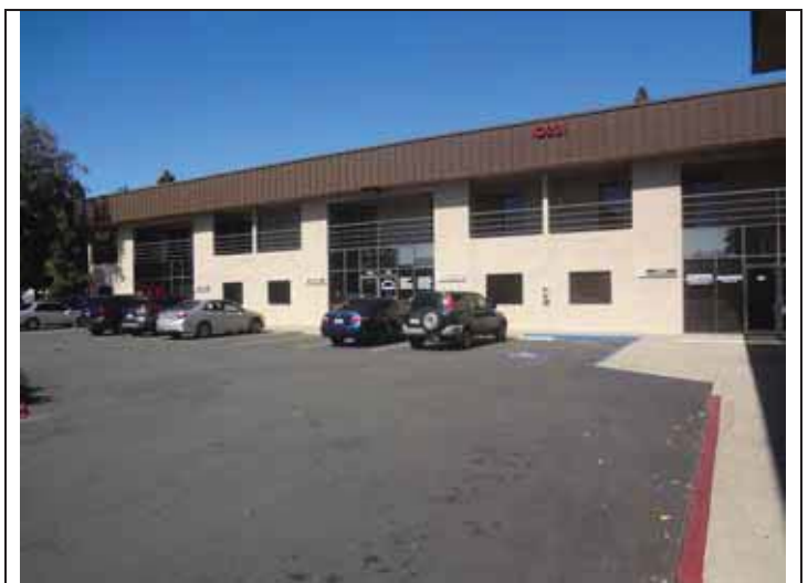
6. South elevation of the 10231 Building.
