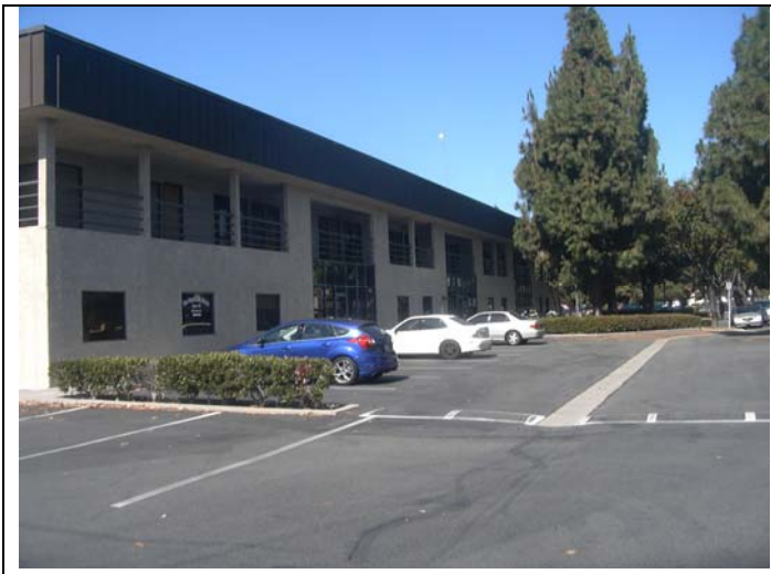
9. View of north side of 10231 building.
