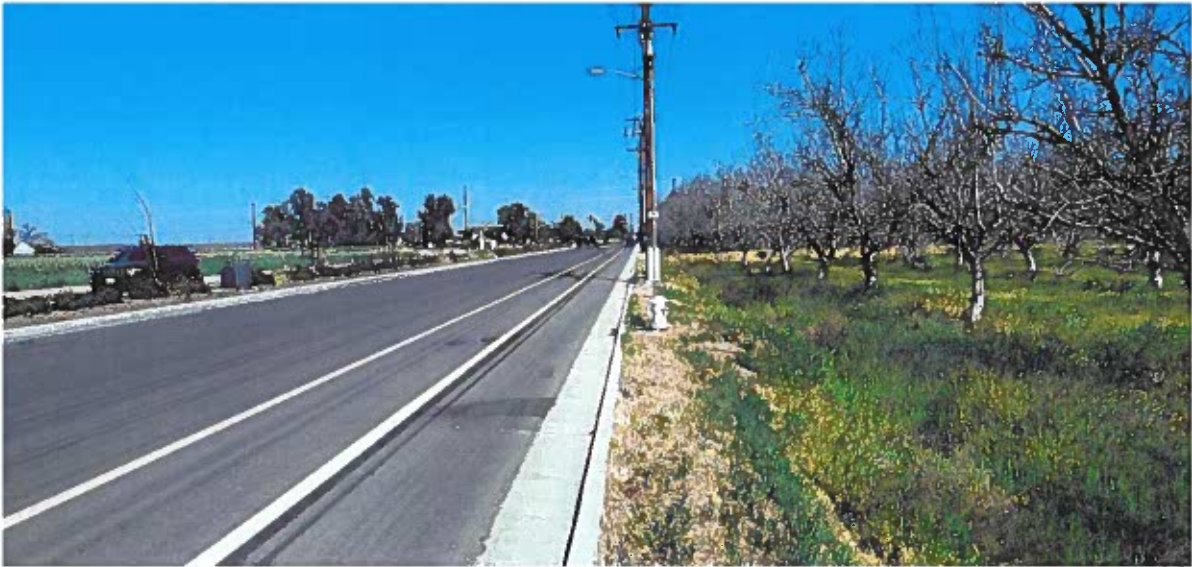
Photo 7: View of the 13 th Ave along west side of Project site.
