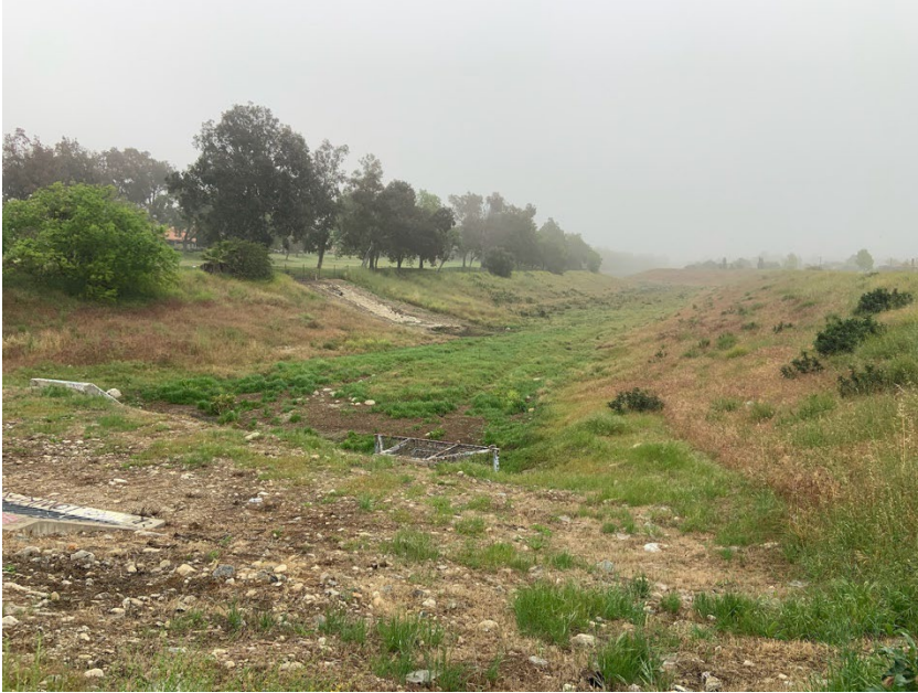
Photo 1. Large culvert near the Western end of the site, facing east.
