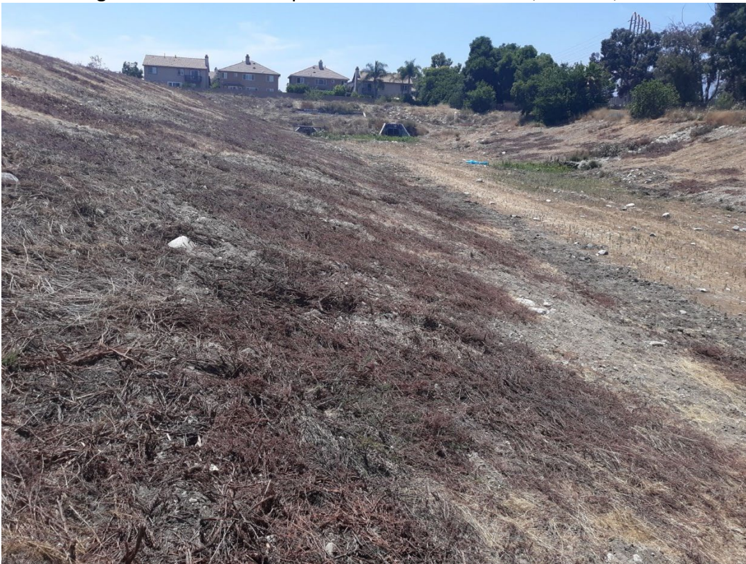
Coastal Sage Scrub habitat at Upland Flood Control Basin after being destroyed by bulldozers, June 23, 2020
