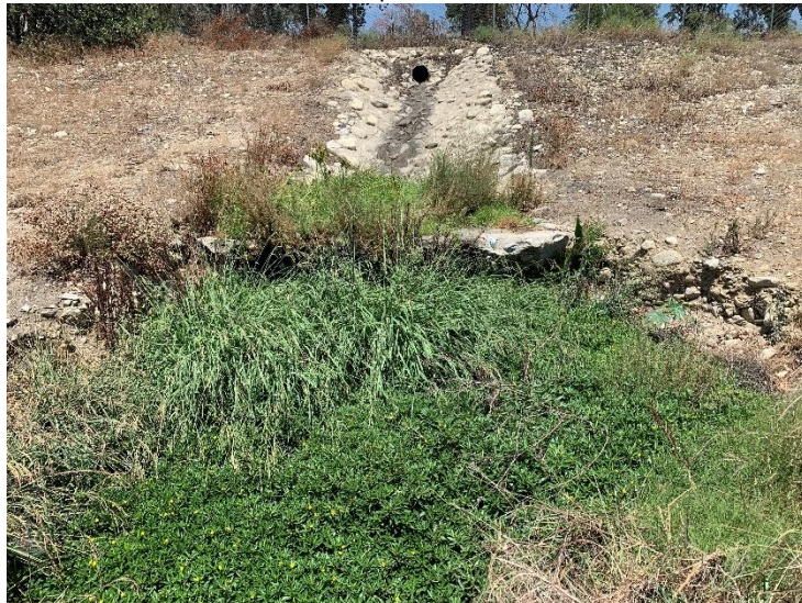
Photo 3: North-facing view of Drainage 2 within the Development Area.
