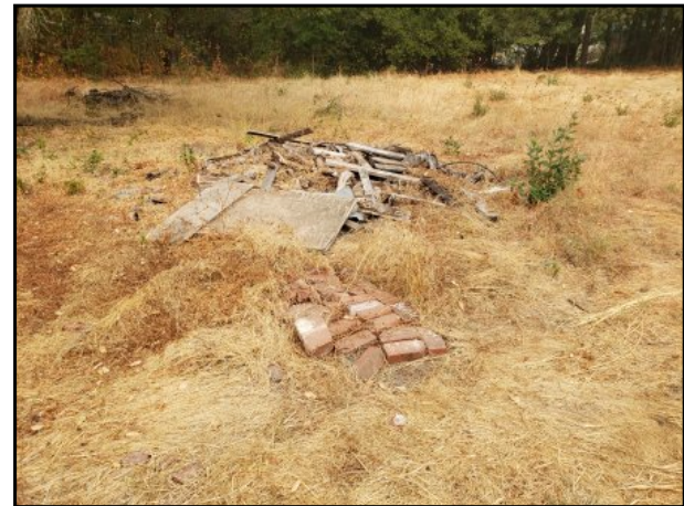
20 : Photograph of demolition debris from former structure located in west section of subject property.
