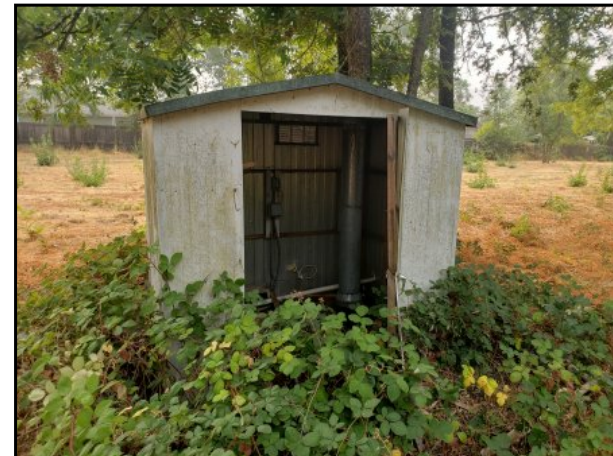
12 : Photograph of sheet metal shed structure located northeast of the wood shed & garage structures.
