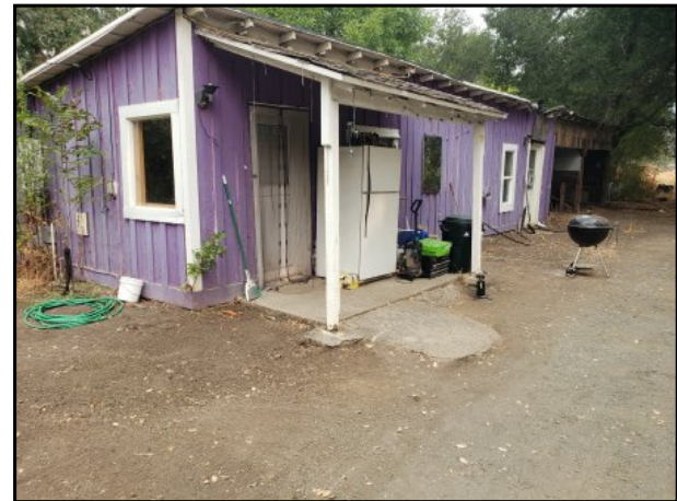
4 : Photograph of wood residential dwelling and attached wood garage.
