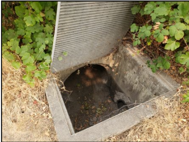
15 : Photograph of storm drainage area with screen located in northwest corner of subject property.
