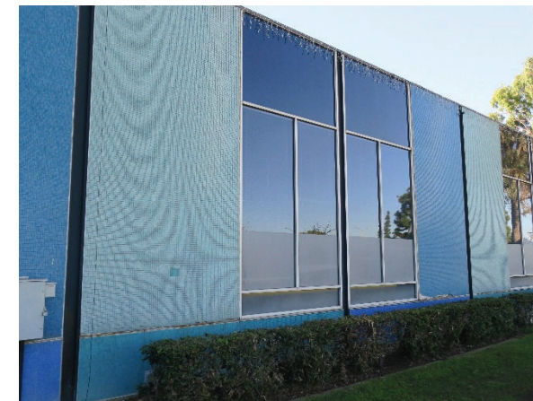
North façade, detail of wall tiles and aluminum windows (ARG, 2022)
