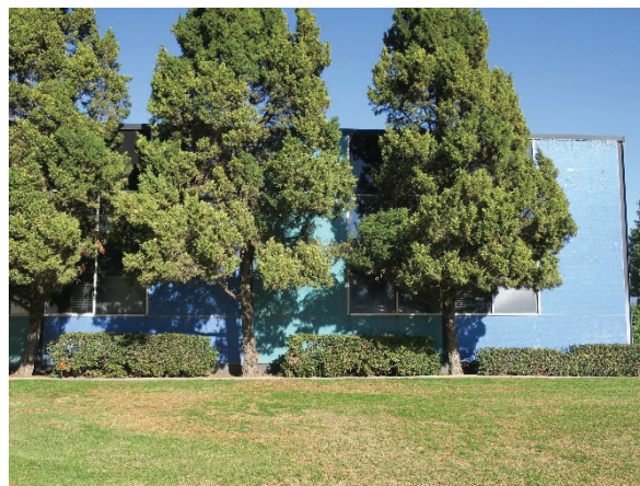
South façade, view north (ARG, 2022)
