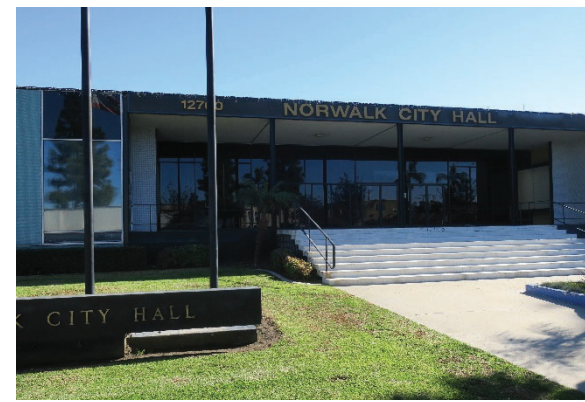
Primary (west) façade, view southeast (ARG, 2022)
