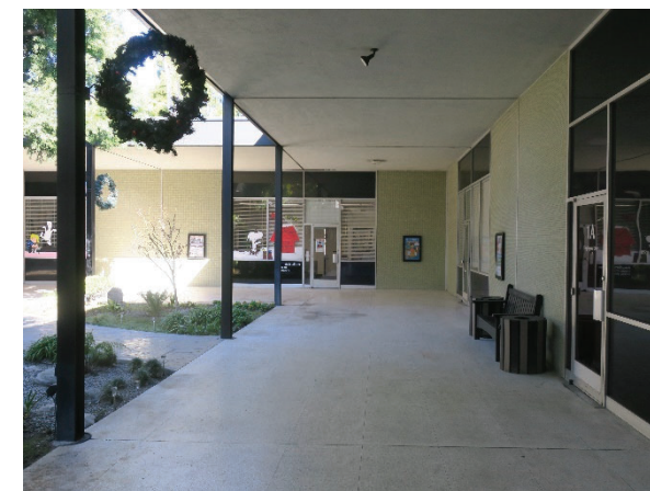
Building viewed from courtyard, view north (ARG, 2022)
