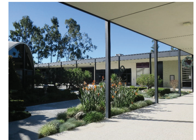
Building viewed from courtyard, view northwest (ARG, 2022)
