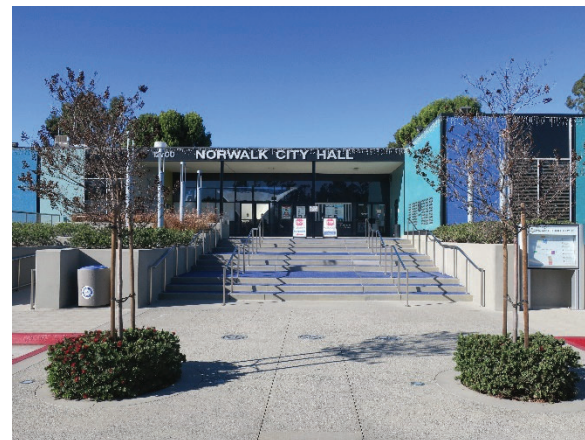
Rear (east) façade, view west (ARG, 2022)
