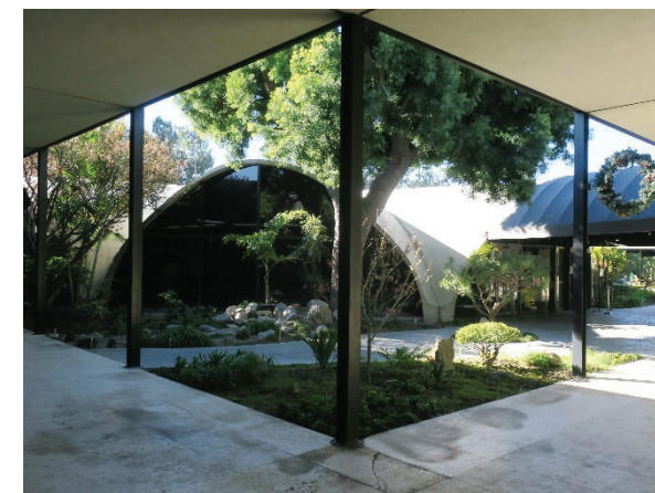
Circular volume at center of courtyard, view southwest (ARG, 2022)
