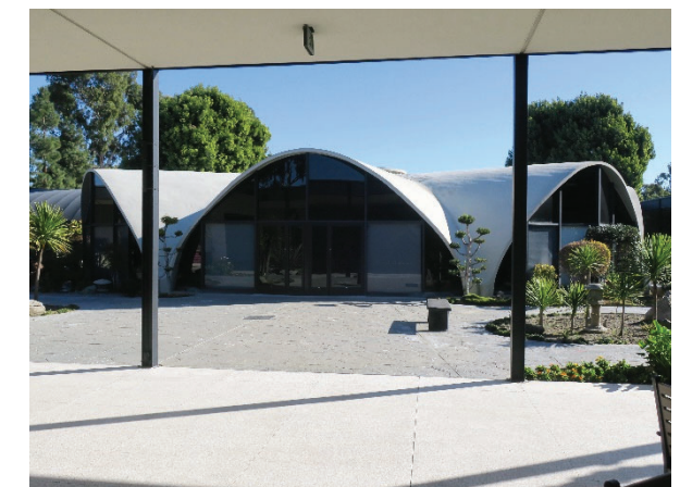
Circular volume at center of courtyard, view northeast. Note ribbed parabolic roof (ARG, 2022)
