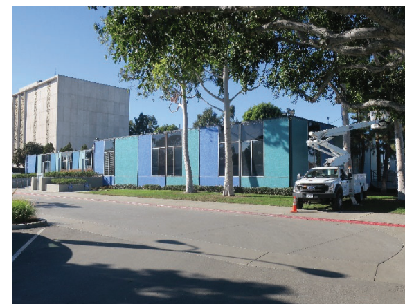
Rear (east) façade, view southwest. Note addition in foreground (ARG, 2022)
