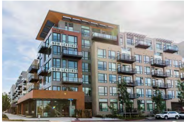
Example of a precedent project in the San Antonio Precise Plan - 400 San Antonio Road
