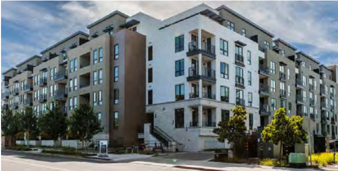
Example of a precedent project in the El Camino Real Precise Plan - 2700 West El Camino Real
