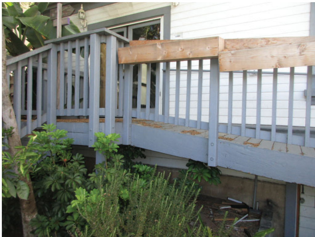
Figure 3-16: Looking northeast at the non-historic OSB board ramp and landing with wood railing. The wood components are termite damaged.
