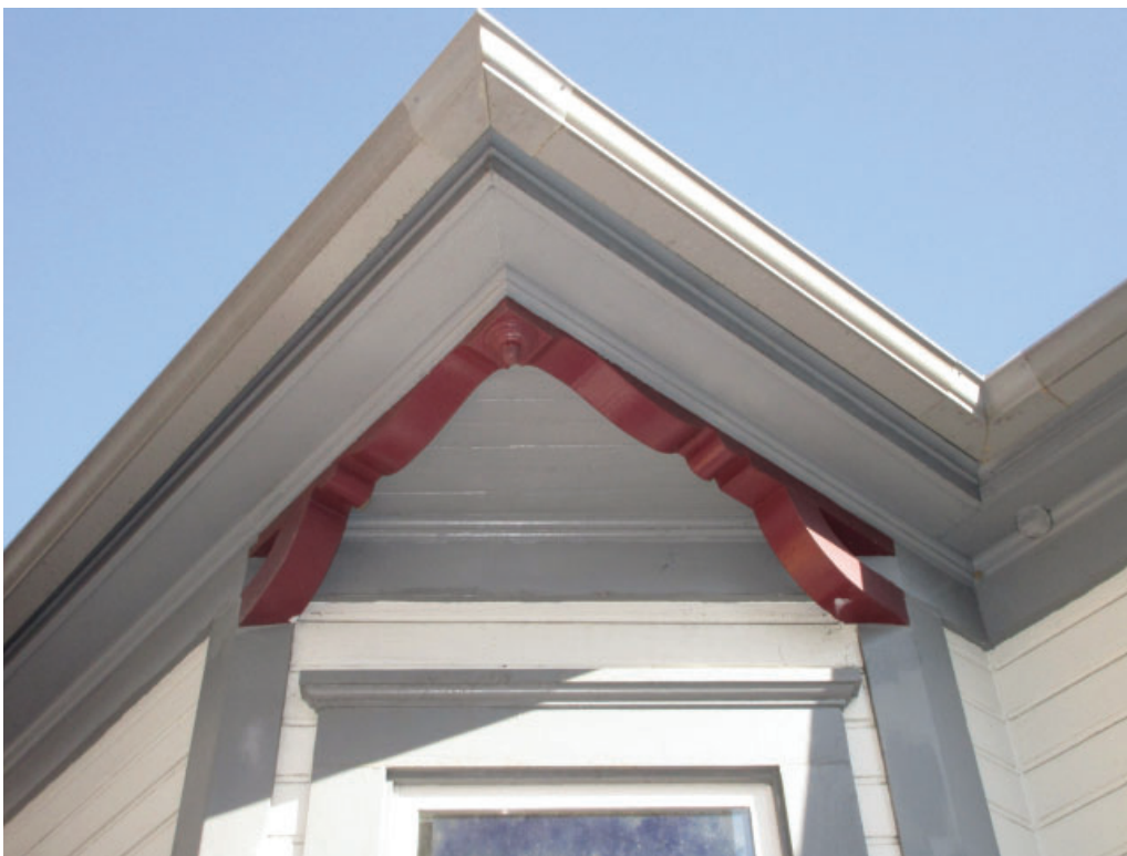
Figure 3-12: Detail photo looking northwest at the projecting roof overhang on the south facade with decorative carved brackets.
