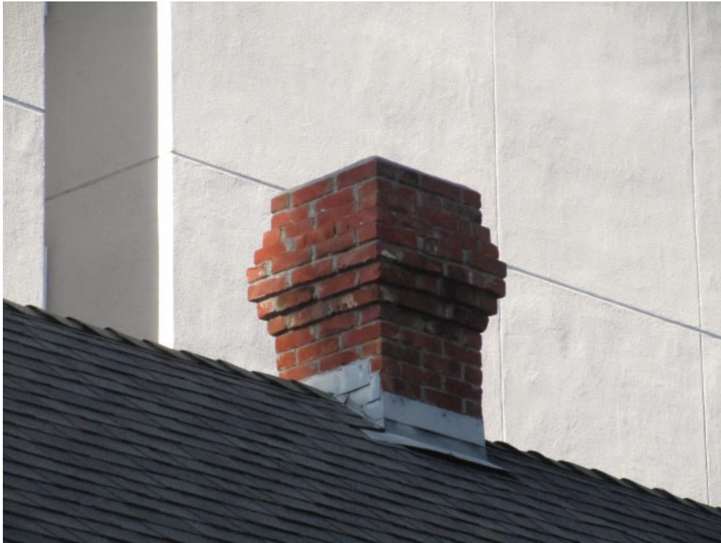
Figure 3-11: Looking southwest at the brick chimney with decorative corbelling.
