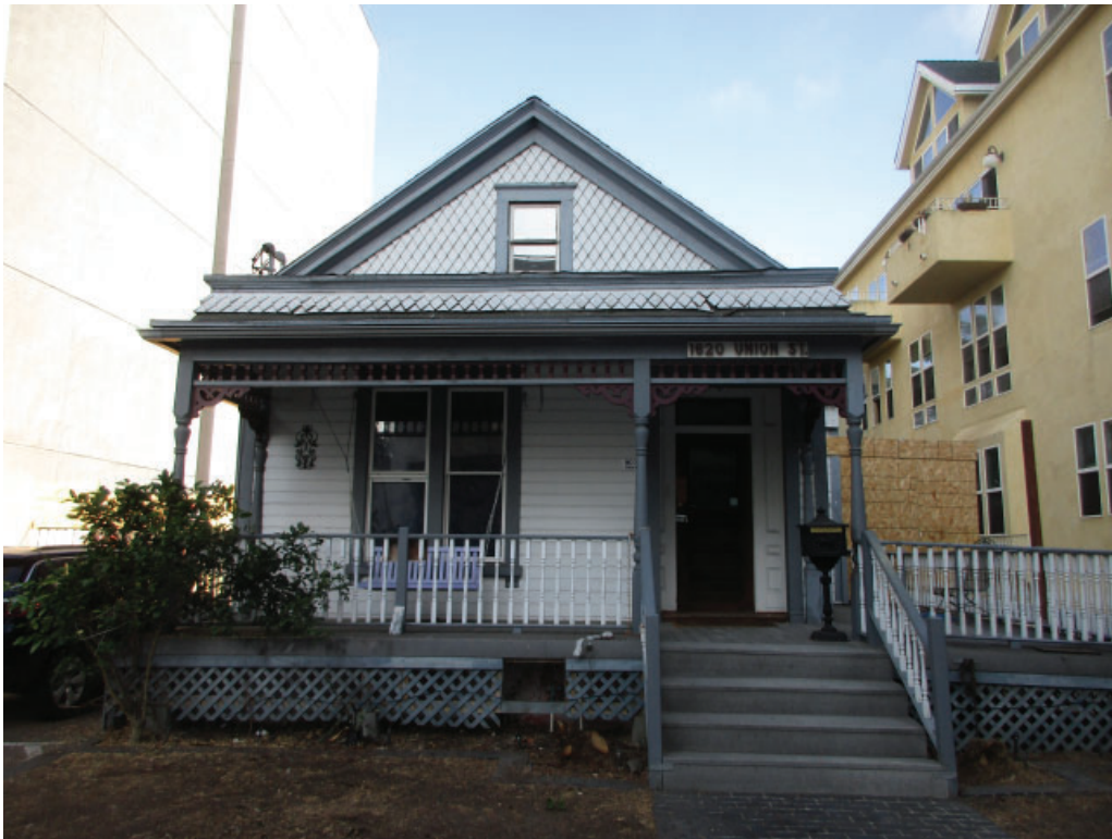
Figure 3-5: Looking west at the primary east facade.
