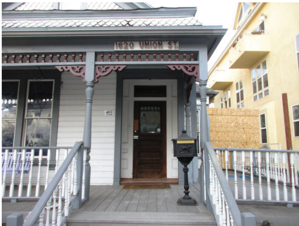
Figure 3-8: Looking west at the decorative porch columns.
