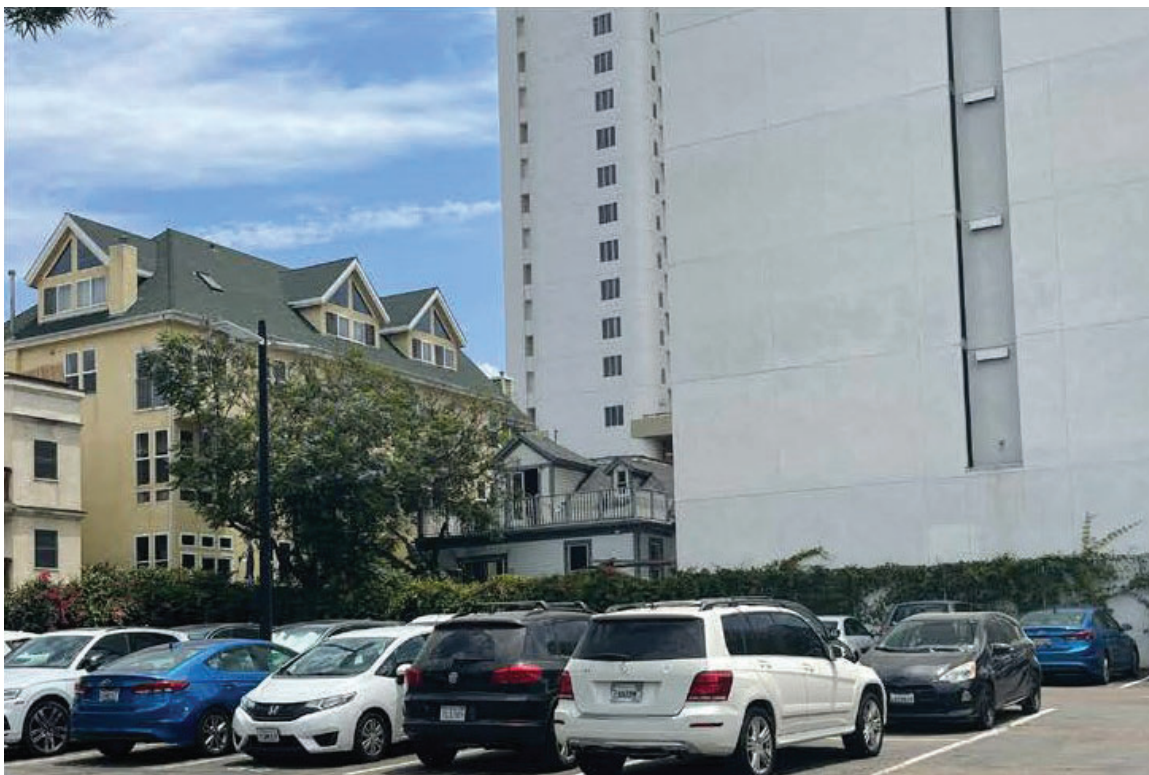
Figure 5-4: Looking northeast at rear of the Andrew Cassidy Home located between two multifamily residences. Source: Matthew Segal.
