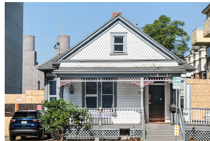
5 PHOTO OF EAST ELEVATION TP-1
