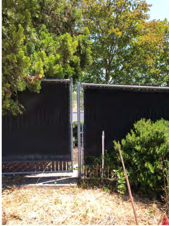
Photo 19 – Stubbed PVC pipe, near east gate
