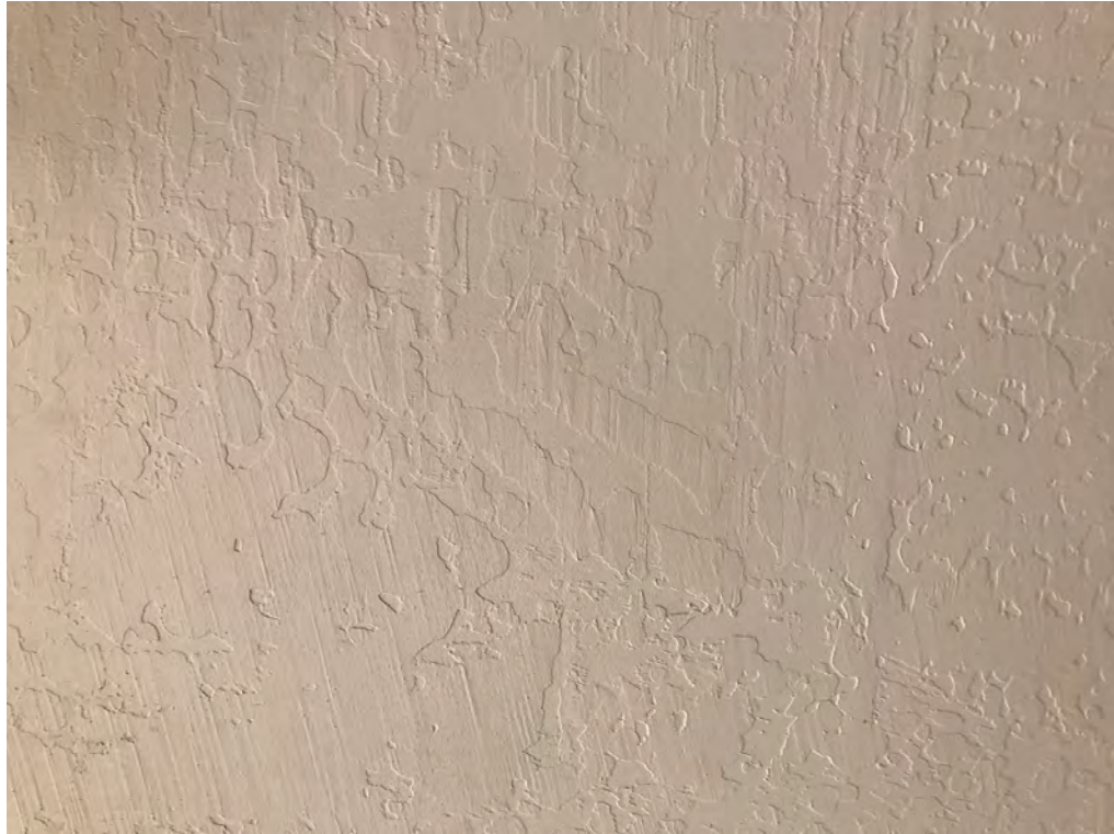
Photo 7 – House, ceiling 2nd floor
