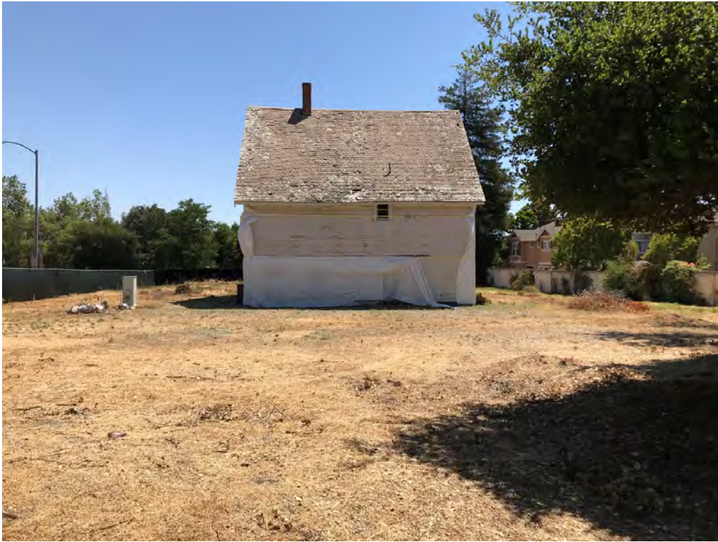
Photo 13 – View of house, looking east from west fence
