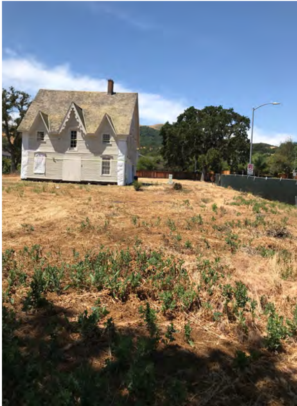
Photo 20 – View of house from north east corner looking west
