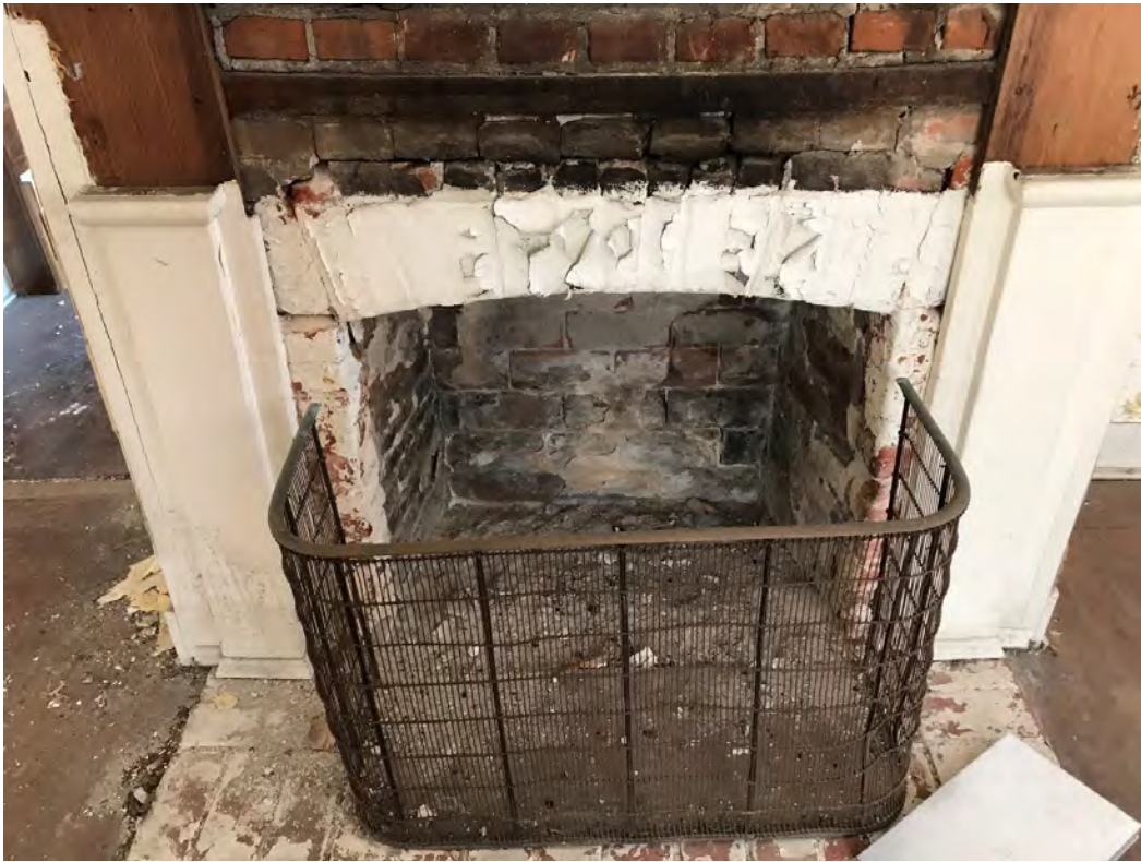
Photo 9 – House, fireplace, 1st floor
