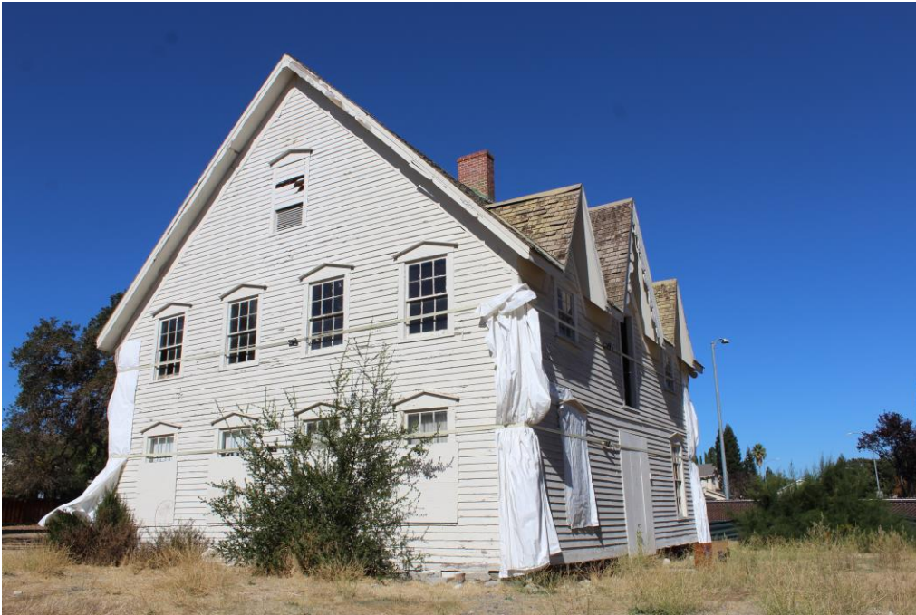
Figure 2: El Nido, north and east façades 14 October 2020.
