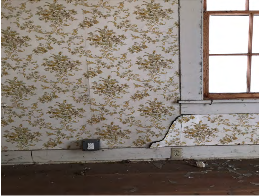
Photo 1 – House, west wall, 1st floor
