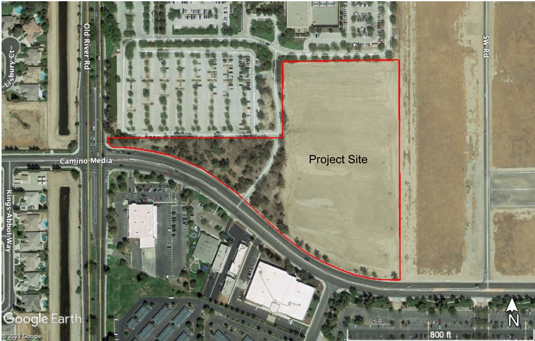
Figure A-2. Aerial photograph of the project site (Google Earth Pro 2021).
