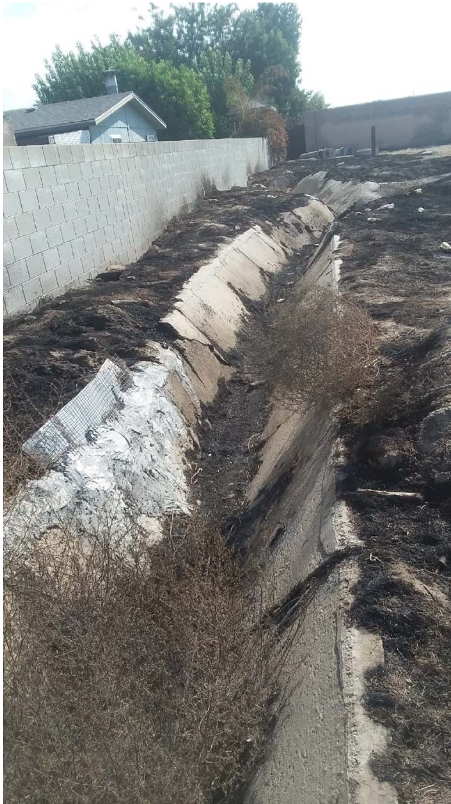
Figure 4 Site M-1, View to the East
