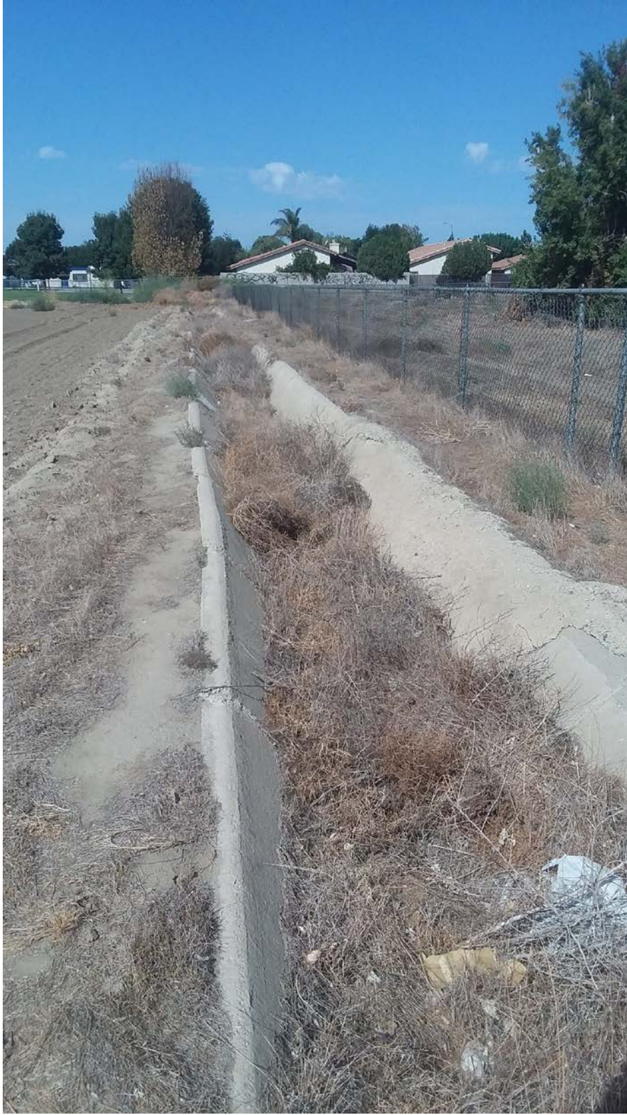
Figure 5 Site M-1, View to the West
