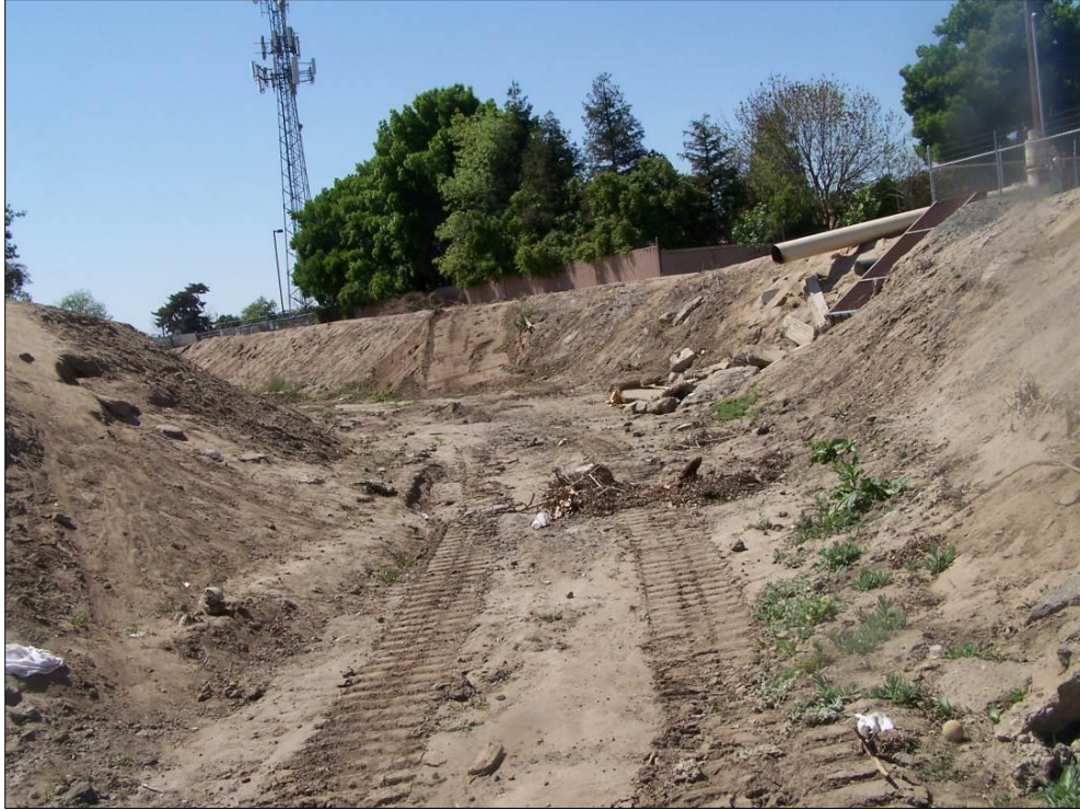
Photo 1: Packwood Creek looking downstream from proposed culvert installation location.
