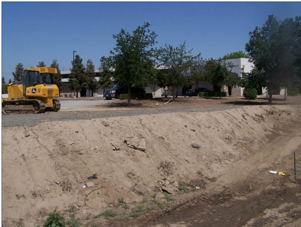
Photo 2: Packwood Creek looking upstream from proposed culvert installation location.
