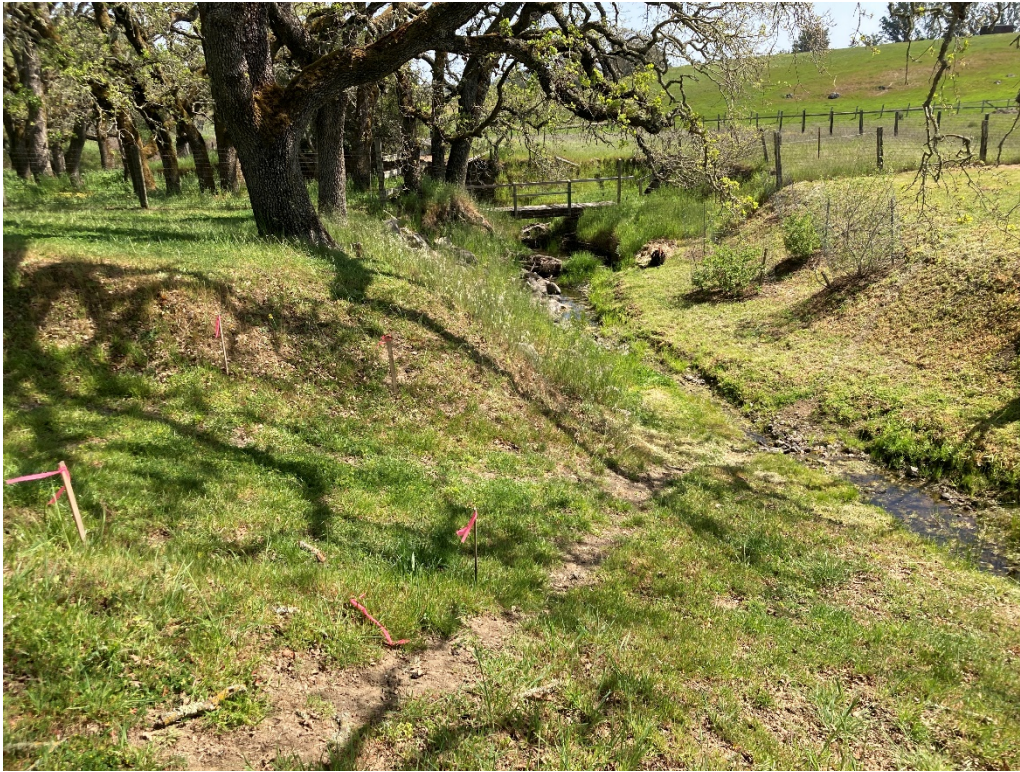
Photo 3. Location of northwestern bridge abutment, existing roadway lacking complex habitat features (April 2022).
