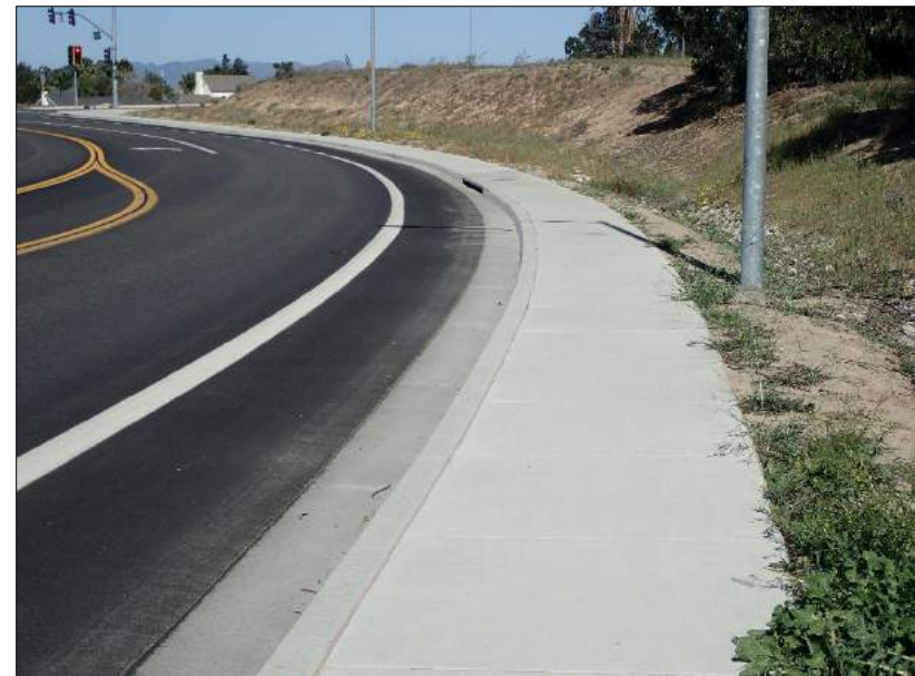
Photo 20: View north rocky roadside drainage ditch & stormdrain inlet along Orcutt Road towards intersection and culvert under UVP. 3/7/2022
