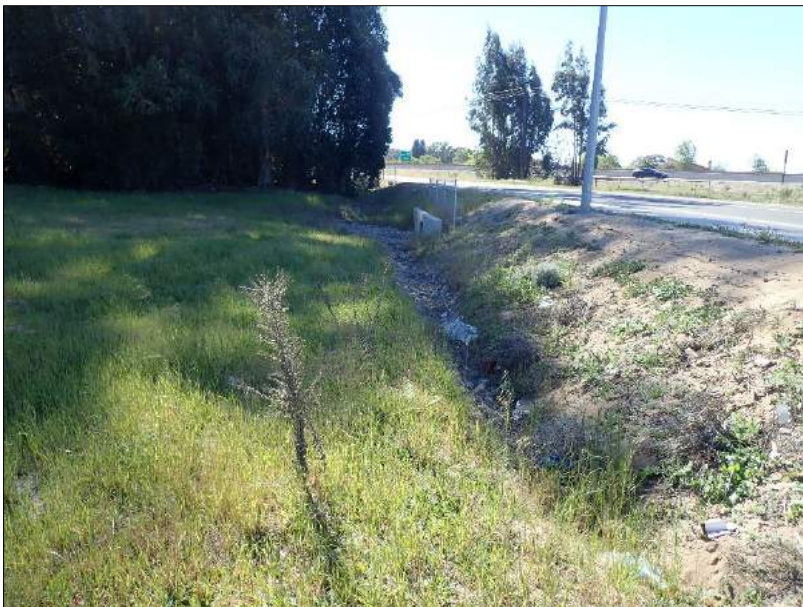
Photo 19: View south at constructed rocky ditch drainage to culvert under Orcutt Road to DP-3 area. 3/7/2022
