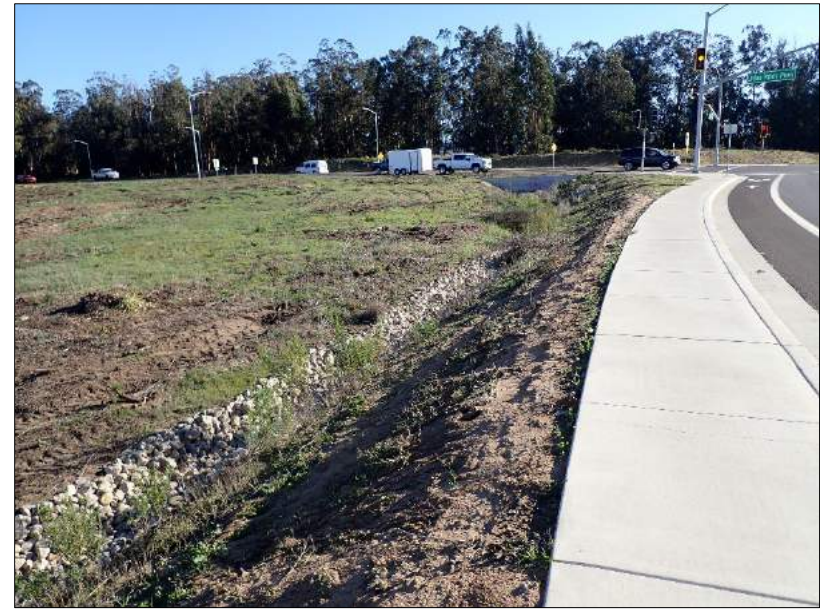
Photo 22: View south at constructed rock ditch roadside drainage management system on Orcutt Road at UVP. 12/17/2021
