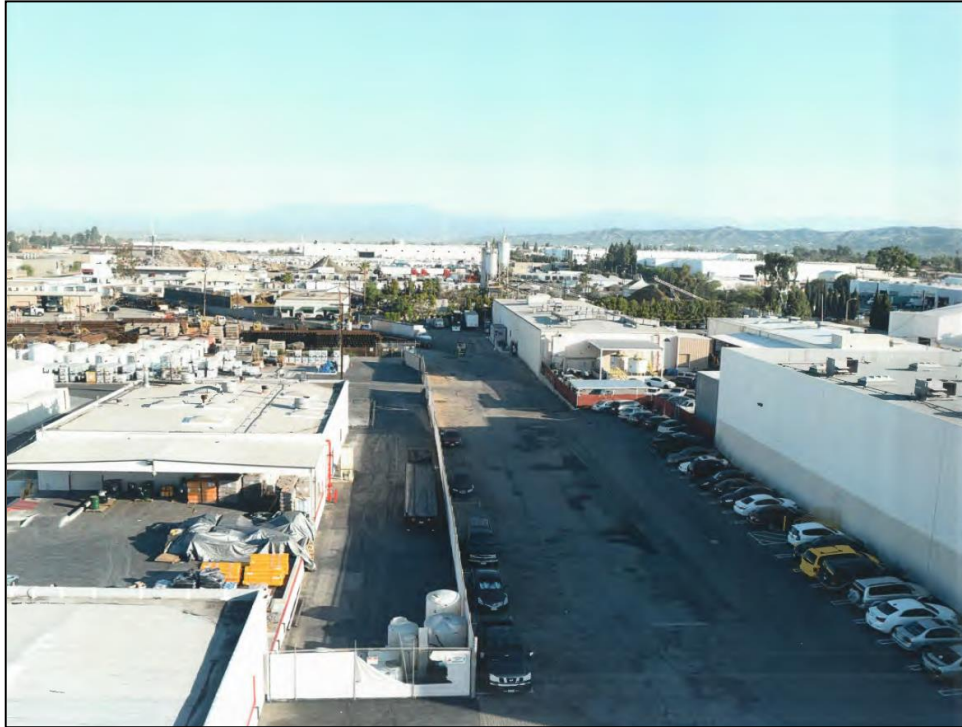
Aerial view of project site driveway, facing north
