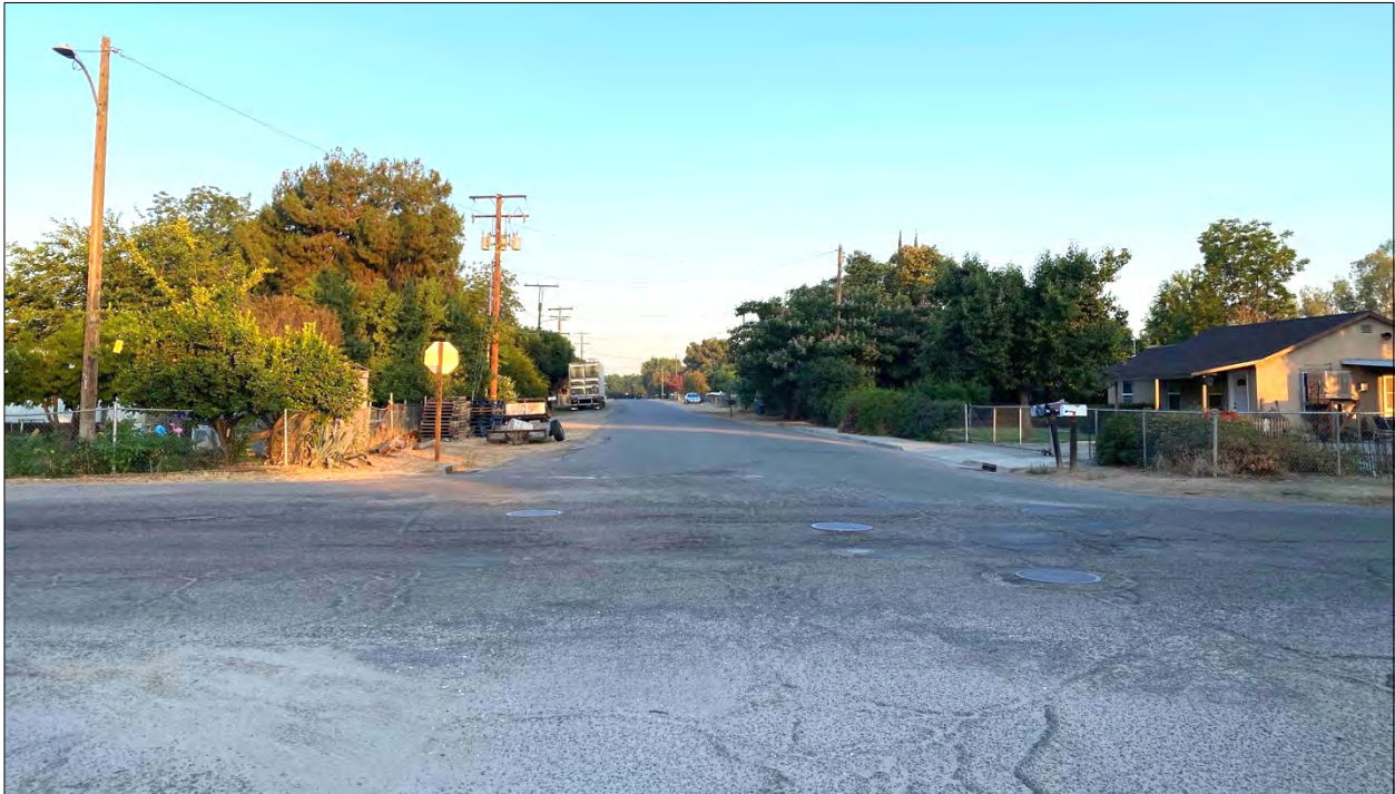
Figure 9. Photograph of the pipeline pathway, looking west along Aspen Avenue, showing the paved roadway, a short, paved sidewalk segment, and surrounding residential development.
