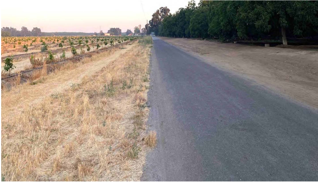
Figure 8: View of the Proposed Pipeline Route along Avenue 324, Looking West, with Immature Citrus Orchard to the South and Mature Walnut Orchard to the North
