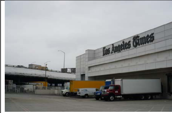
South portion of rear (east) façade, view southwest (Atlas, 2020)
