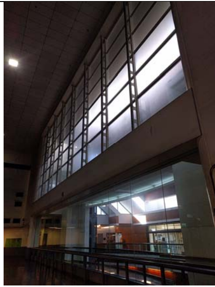
Glazing separating press room/reel room from main lobby, view southwest from press room
