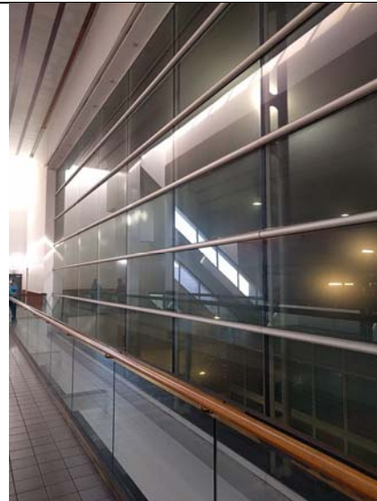
Glazing separating press room from main lobby, view northeast from lobby walkway
