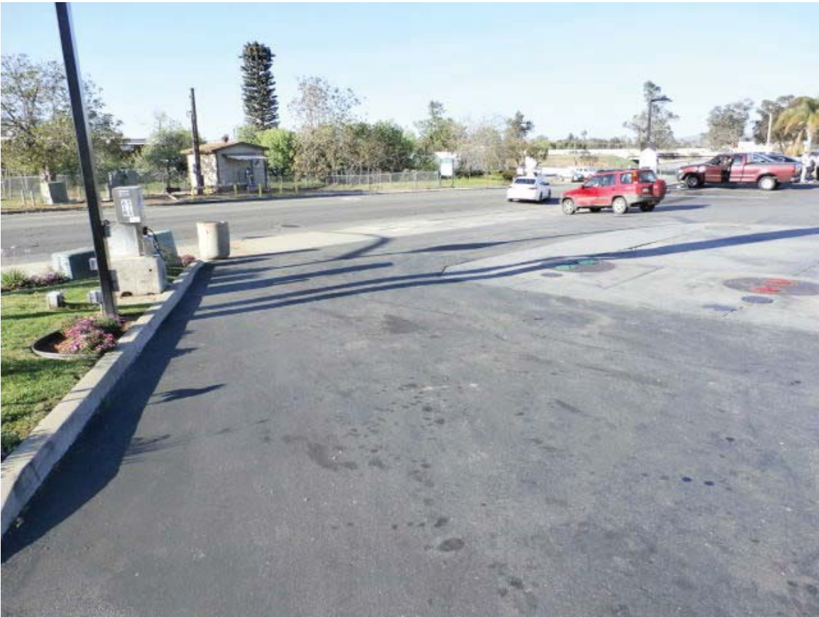
PHOTO 5 - VIEW OF THE UNDERGROUND STORAGE TANKS (USTs) AT THE FASTRIP GAS STATION ON THE RIGHT. THE CURB TO THE LEFT IS THE APPROXIMATE EDGE OF THE PROPOSED IMPROVEMENTS ON THIS CORNER, LESS THAN 20 FEET FROM THE EXISTING USTs. IN THE BACKGROUND, ACROSS THE STREET TO THE LEFT, IS THE SOUTH MESA WATER COMPANY WELL #11 SITE.
