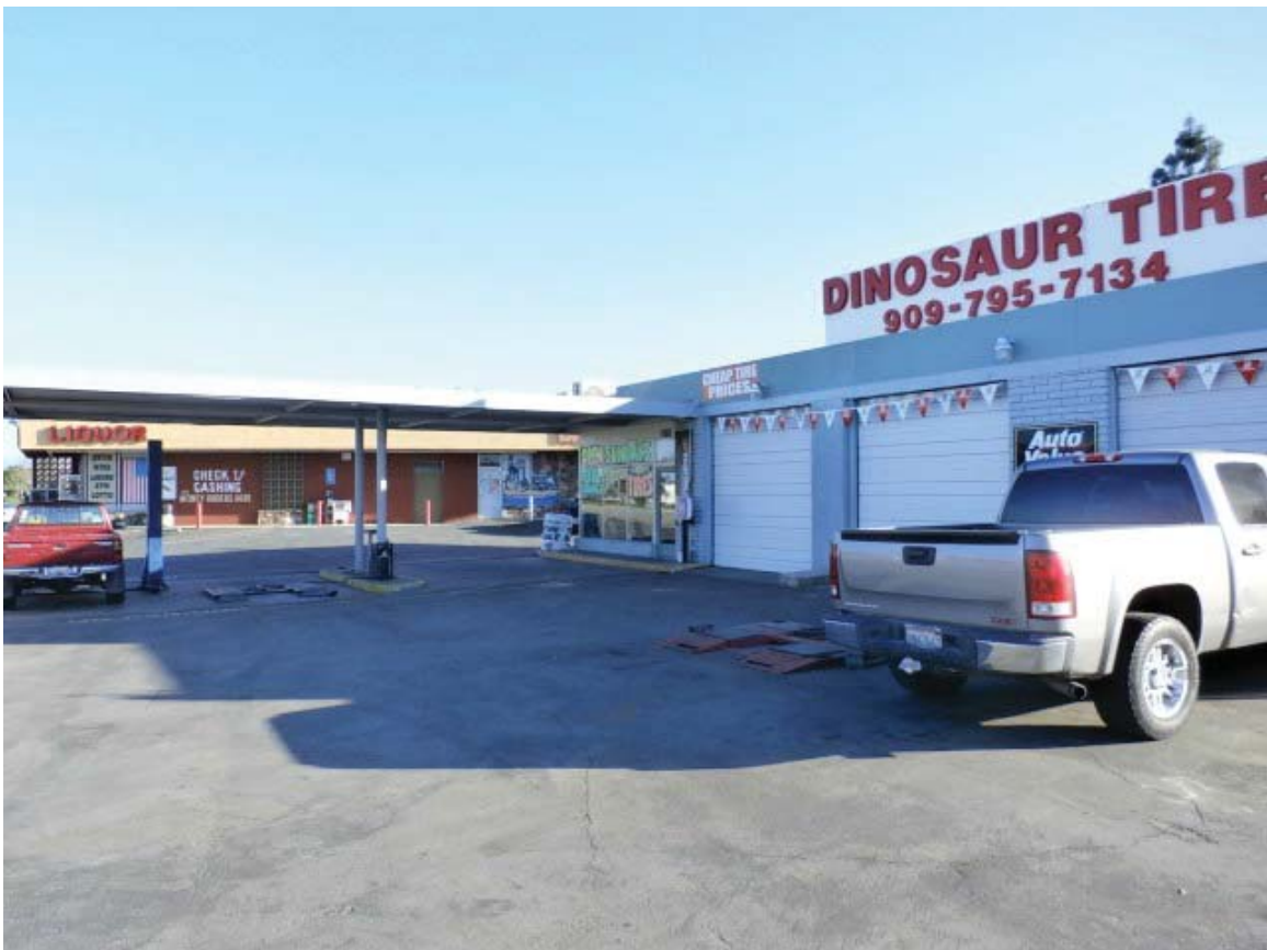
PHOTO 2 - VIEW FACING NORTH, SHOWING THE DINOSAUR TIRE CENTER AT 13715 CALIMESA BOULEVARD, WHICH IS SCHEDULED TO BE OBTAINED UNDER THE PROPOSED PROJECT FOR THE SUBJECT SITE. ONE OF THE FORMER GASOLINE STATION DISPENSER ISLANDS IS VISIBLE UNDER THE CANOPY. IN THE BACKGROUND IS PART OF THE SHOPPING CENTER SHOWN TO THE RIGHT IN THE PREVIOUS PHOTOGRAPH.
