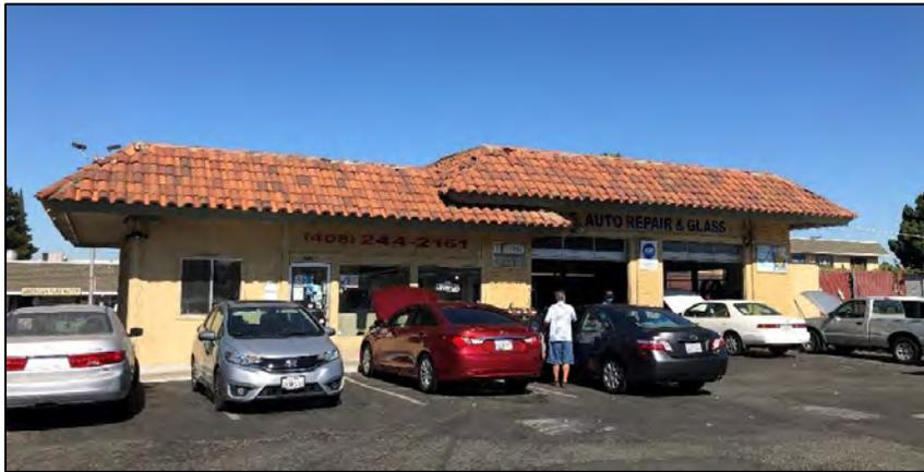
The canopy, which also has a mansard roof with clay tile, shelters the location of the former gas pumps.
