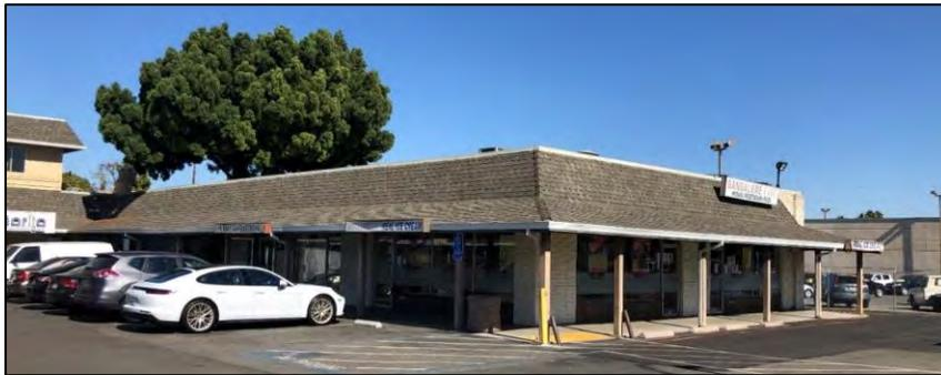
and has wooden board and batten cladding on the walls on the ground floor below the storefront windows. A mansard-like<sup>19</sup> asphalt shingle-clad structure functions as a parapet and hides the flat roof that covers most of the structure at the first floor. An asphalt shingle-clad mansard roof tops the second floor and hides the mechanical units on the roof. The east and north façades of the complex face narrow vehicle access ways which are also used for parking.
