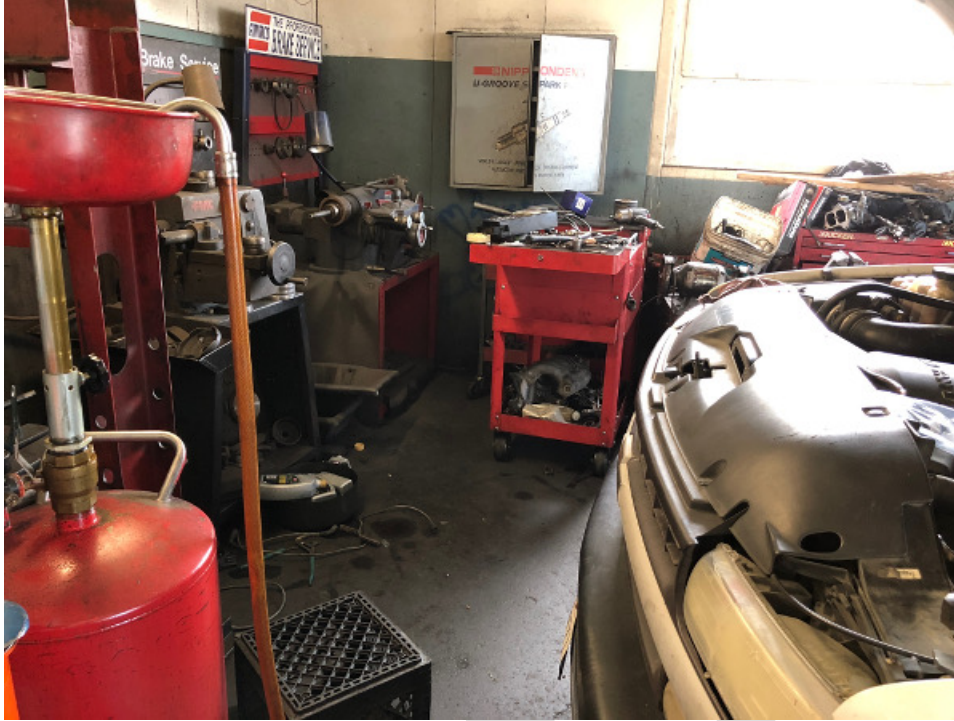
Photograph 66. Sanding / brake service machinery in northeast corner of structure.
