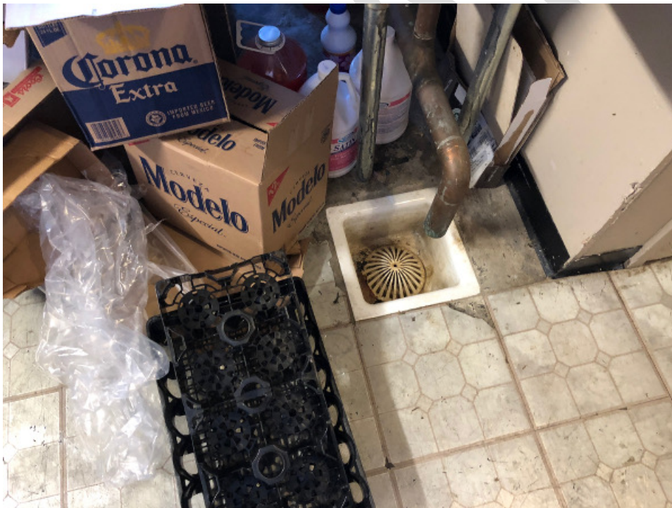
Photograph 16. Floor drain within convenience store unit.
