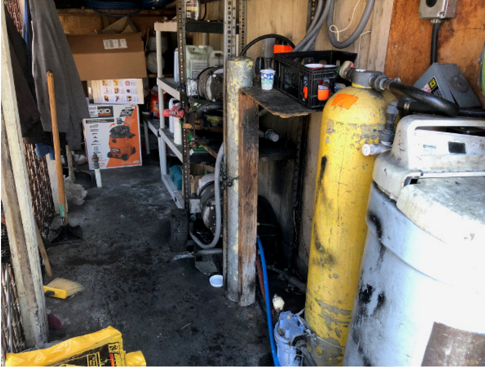
Photograph 79. Car wash related equipment alongside fenced area and car wash office.
