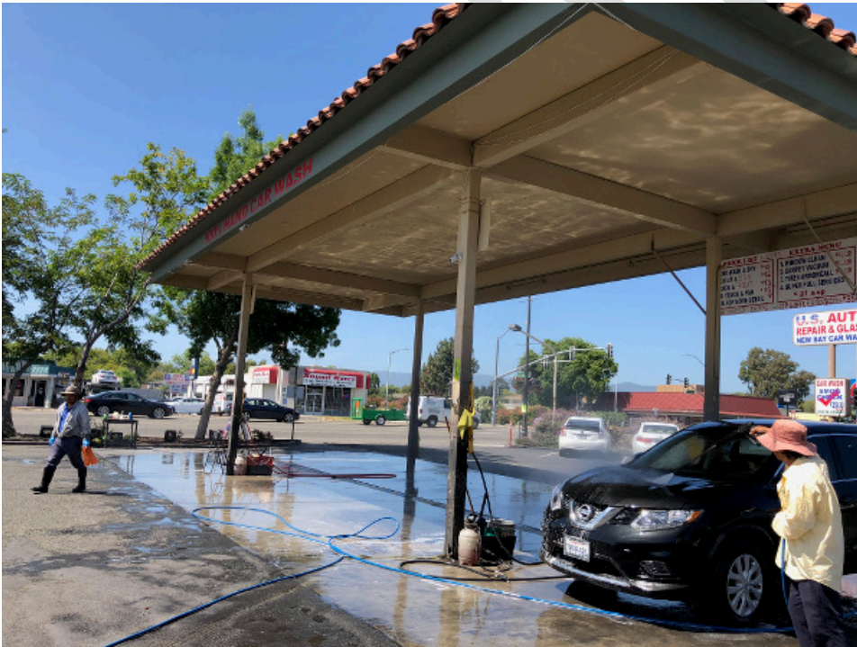
Photograph 61. View looking southwest at car wash awning.
