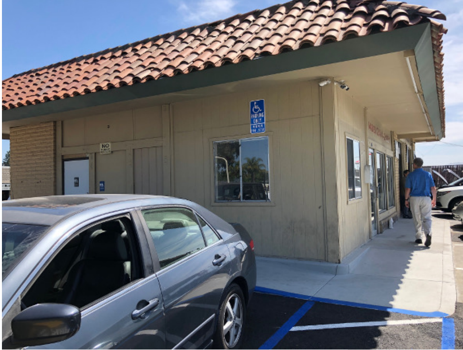
Photograph 62. View looking east at automobile service structure.
