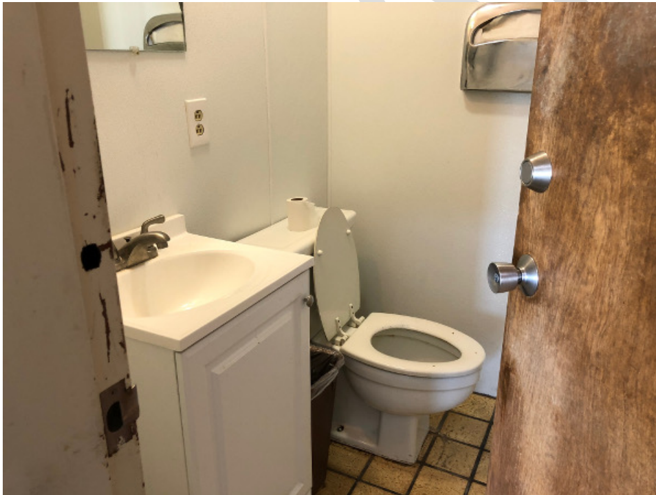
Photograph 30. Typical restroom within ground-floor office lobby.
