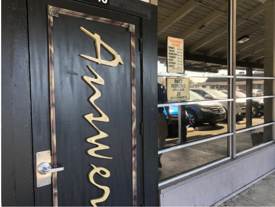
Photograph 17. Exterior of bar / restaurant tenant unit.
