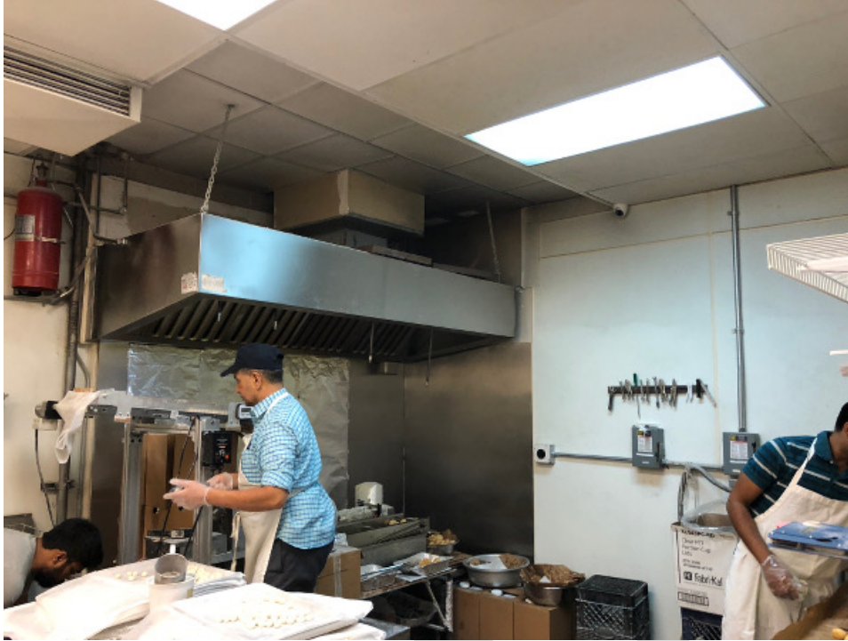
Photograph 9. Additional view of kitchen within bakery tenant unit.
