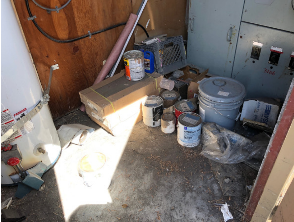
Photograph 52. Additional view of paint and property maintenance supplies.
