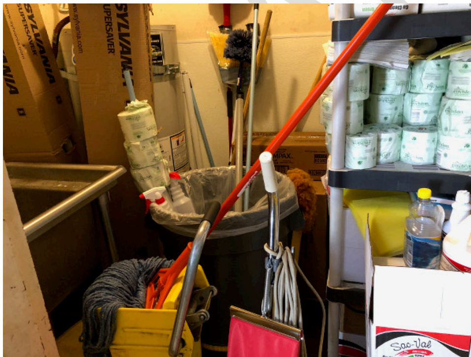
Photograph 28. Janitorial closet within ground floor of office lobby.
