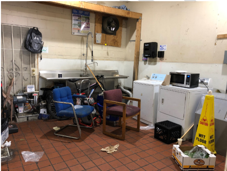
Photograph 42. Washer & dryer, ice machine and sink within rear of additional market tenant space. Washer and dryer reportedly drains to an exterior containment.
