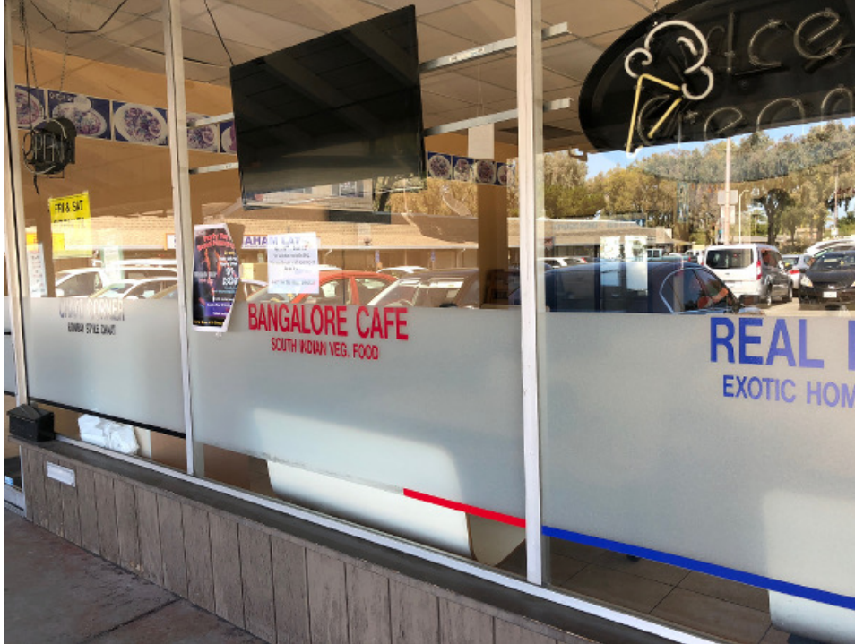
Photograph 48. Exterior of additional restaurant and ice cream shop (unable to enter interior, closed for renovations).
