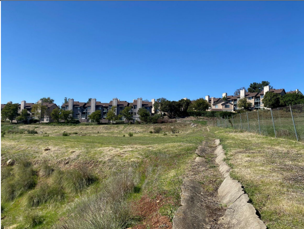
Photograph 4: West-facing view of a concrete stormwater swale outside and north of the project site.
