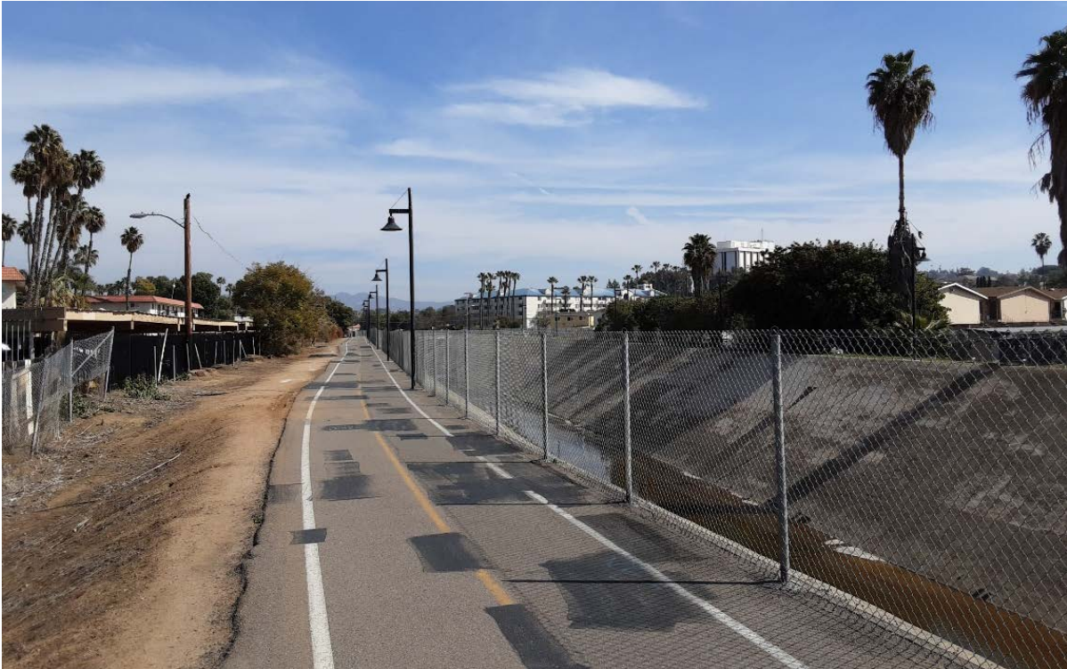
Figure 7 Eastward view of trail corridor and lighting fixtures, to east of N. Broadway
