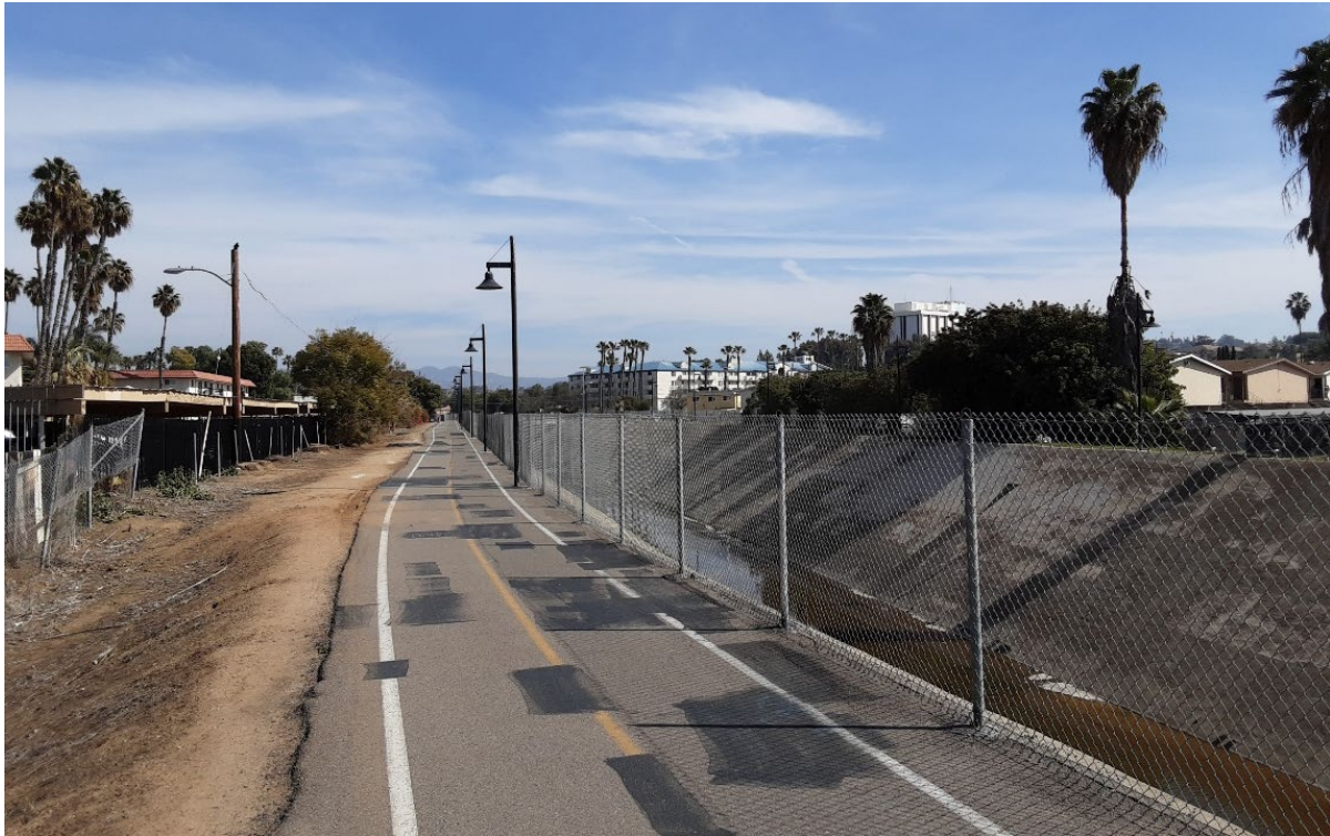
Photograph 7. Eastward view of trail corridor and lighting fixtures, to east of N. Broadway.
