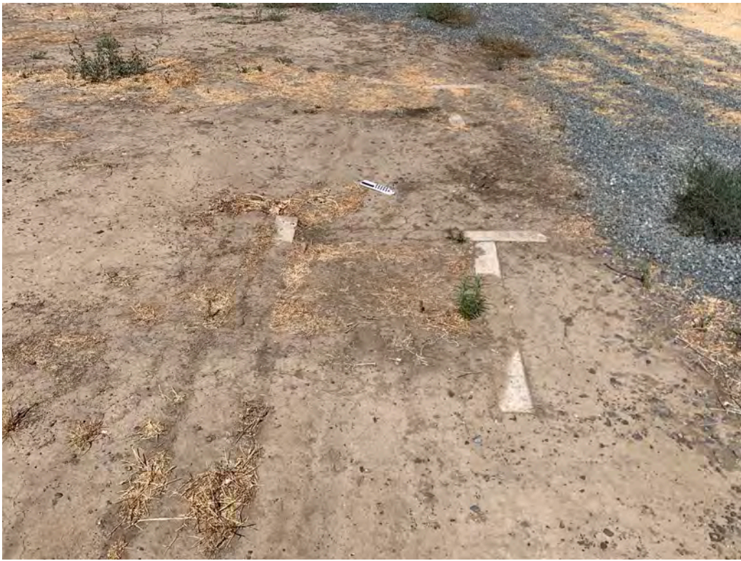
Photo 15: Possible structure footing/foundation remnants, facing west/southwest
