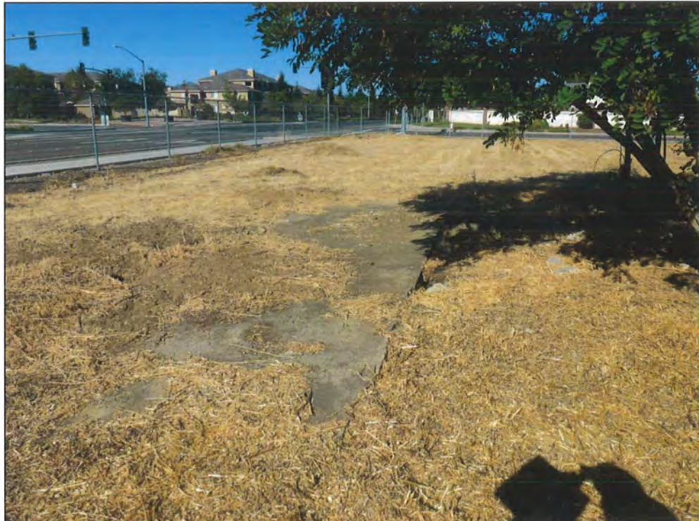
Raised concrete pad overview, view west, 8/23/2013, Photo #011
