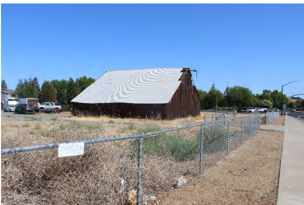
Photograph 5. South barn, view looking north towards Lone Tree Way (Stantec 7/12/21)
