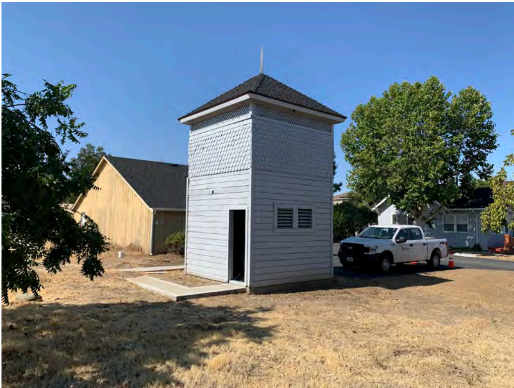
Photo 13: Overview of structure on property, facing southwest
