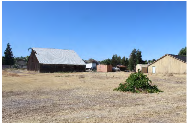
Photograph 4. North and south barn, view looking south (Stantec 7/12/21)
