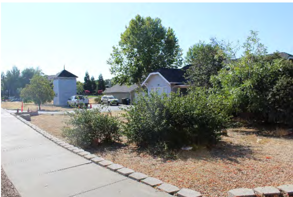
Photograph 2: Project site, view looking east towards residence, tankhouse, and north barn (Stantec, July 2021)
