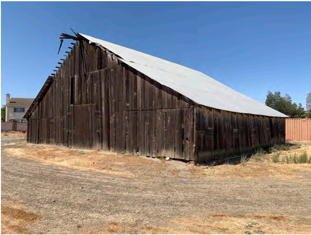
Photo 11: Overview of structure on property, facing southwest
