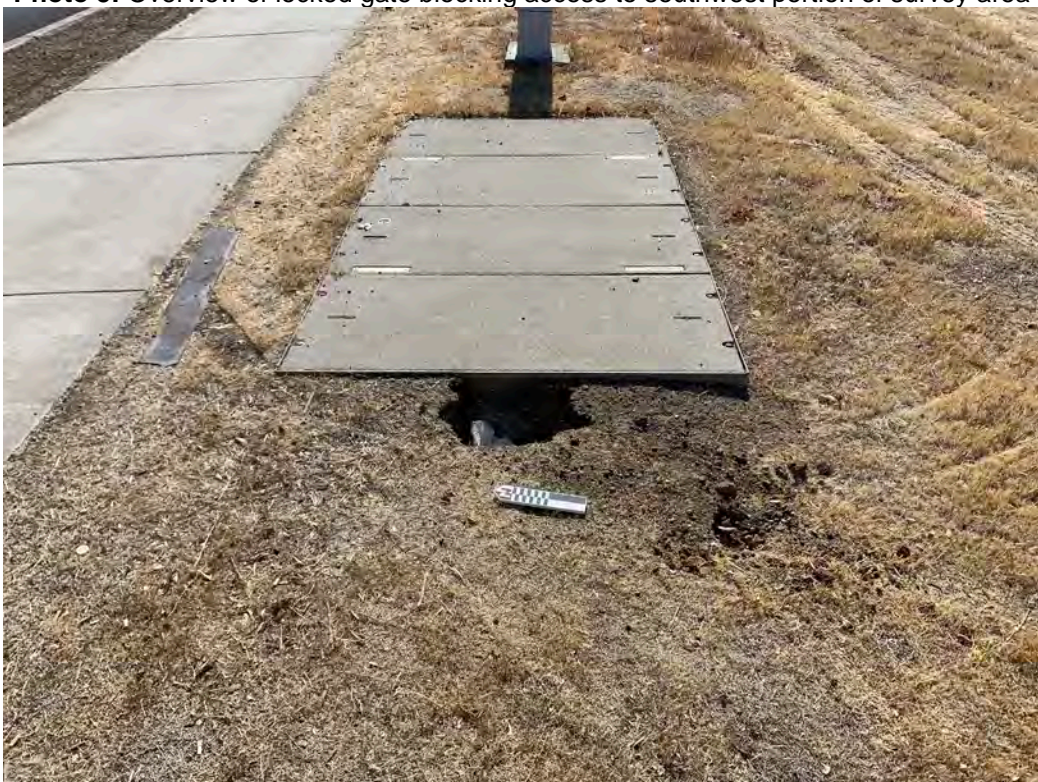
Photo 6: Overview of utilities vault (disturbance), facing east
