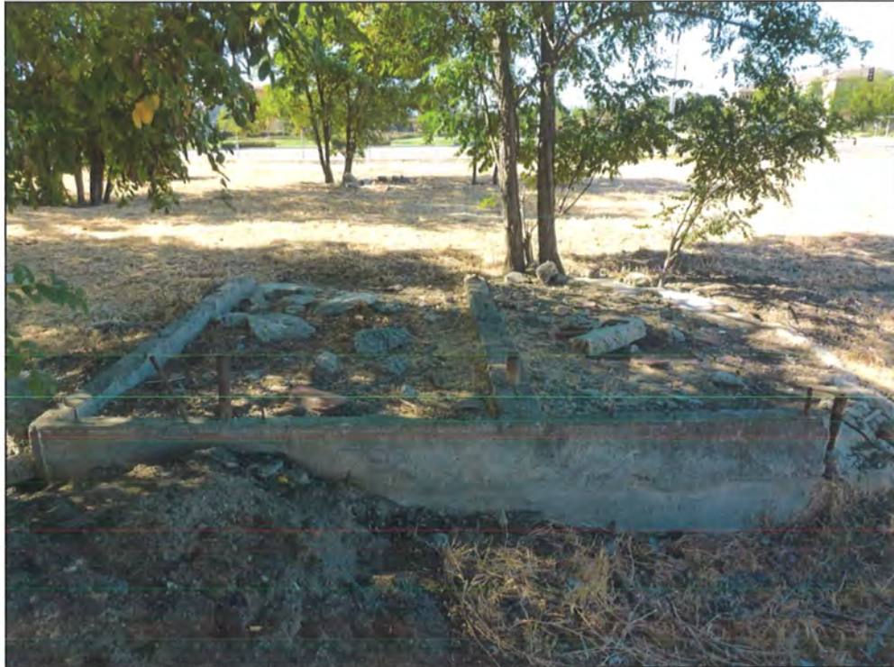
Possible bathroom foundation with raised concrete pad in background, view south, 8/23/2013, Photo #006
