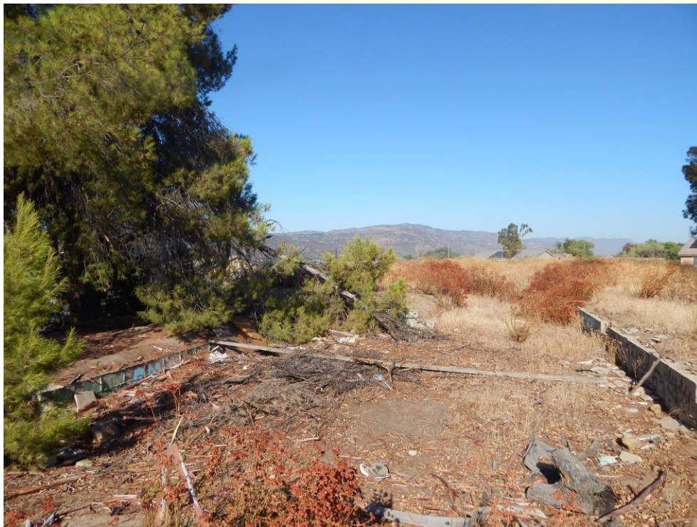
Plate 3. Overview of modern cinderblock foundation. View towards west.
