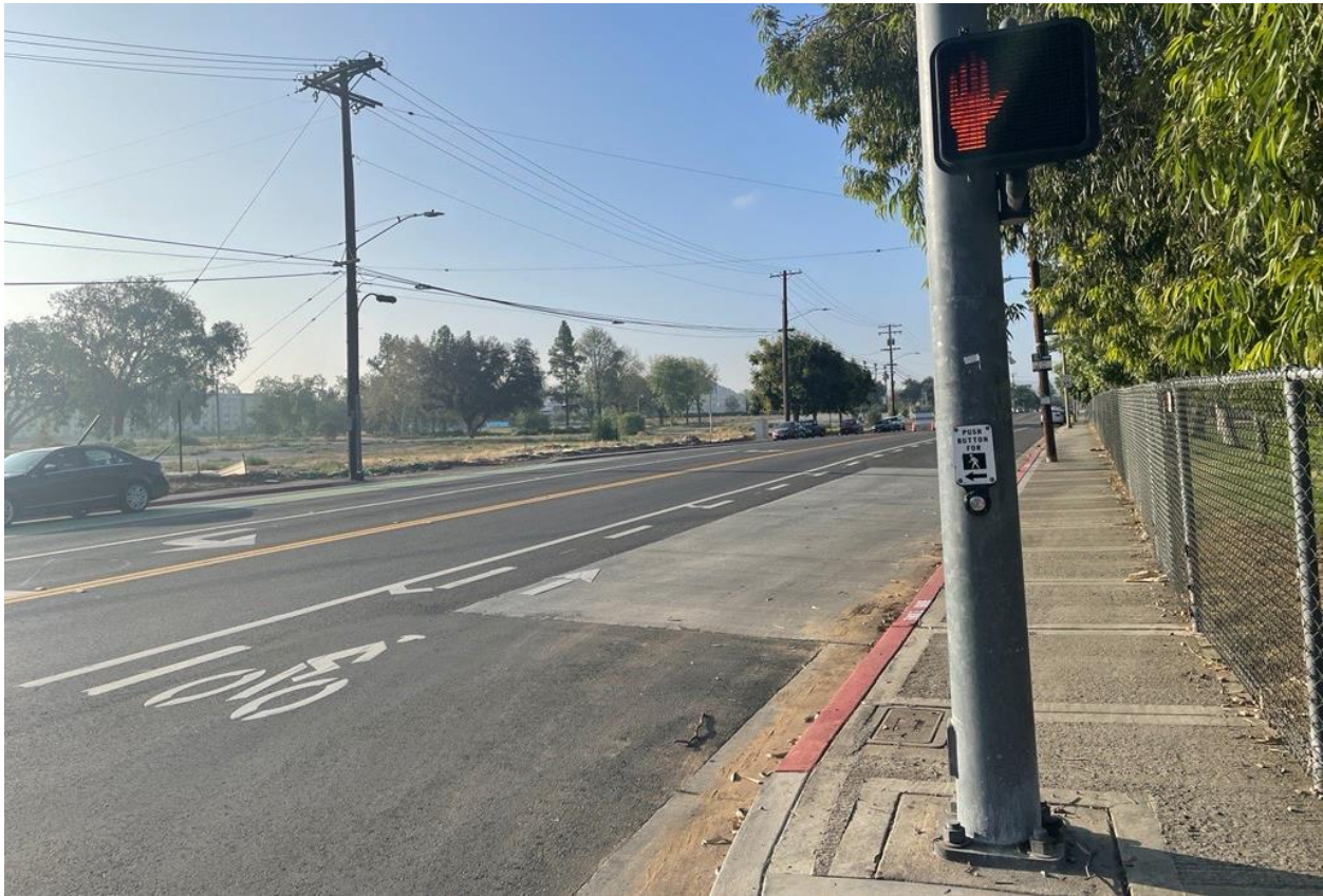
Figure 9 Photo 5 Overview of Electrical Feeder Line Upgrade Alignment (Blaine Street at Rustin Avenue), View to the East
