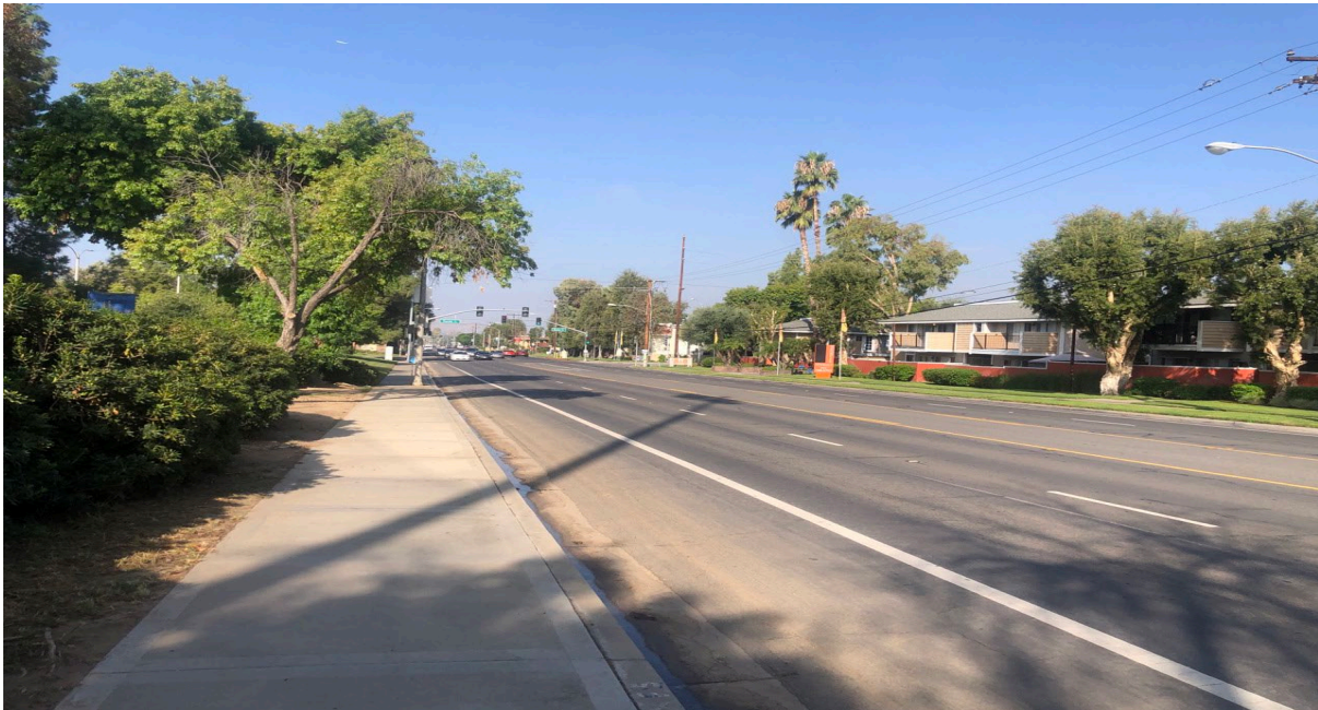
Photograph 4. Proposed electrical feeder line upgrade alignment area along Blaine Street. Taken September 16, 2022.
